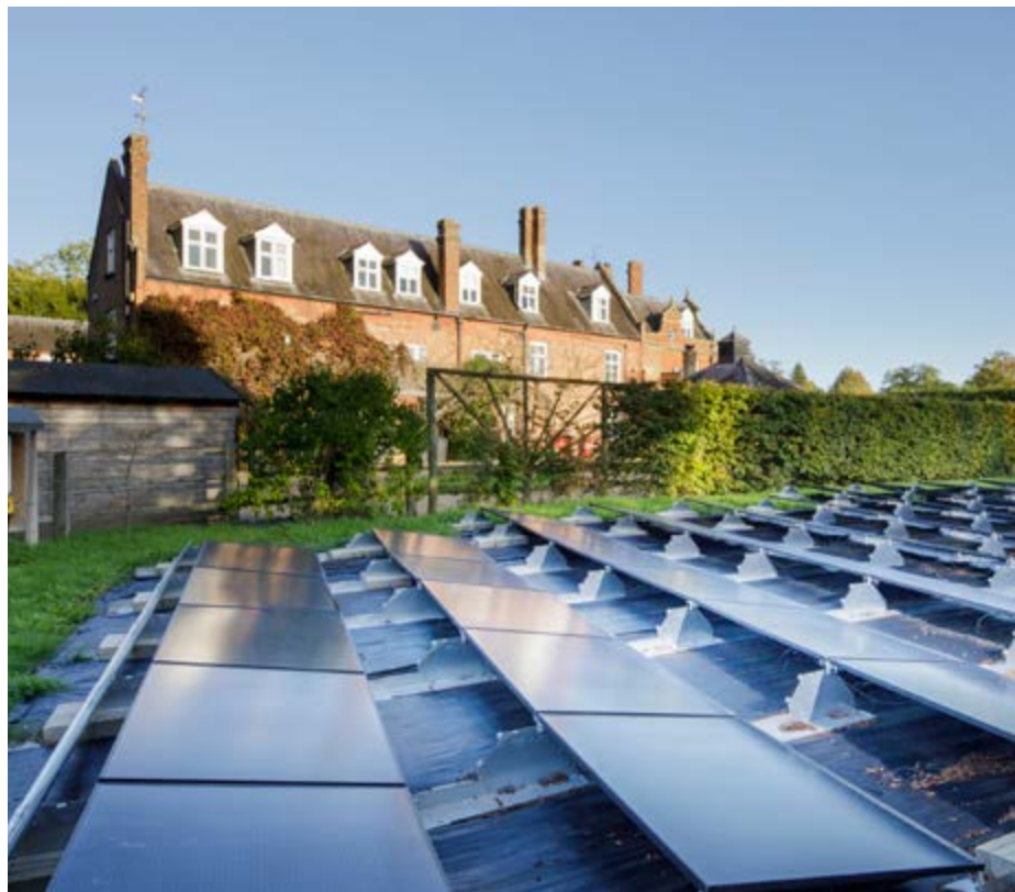
Chippenham Hall, Chippenham, Cambridgeshire. Solar panels have been installed in the garden.
