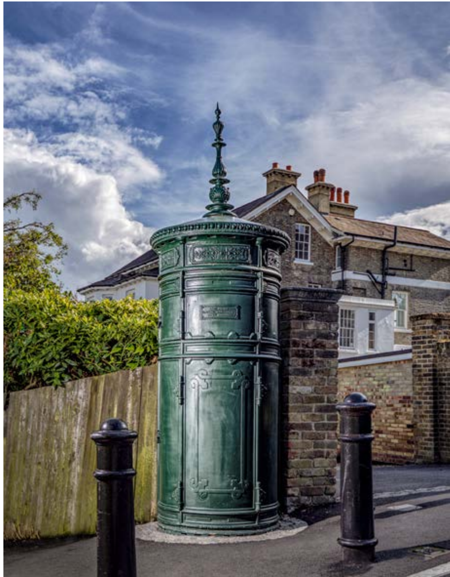
A rare, Victorian electricity substation at Sunnyside, Wimbledon. This was saved and removed from the Heritage at Risk register in 2023.
