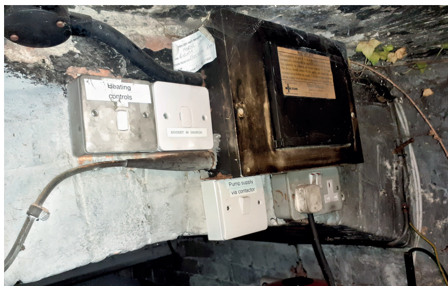
A smoke-blackened consumer unit in the parish church of Bibury, Oxfordshire (Photo: Dan McNaughton)
