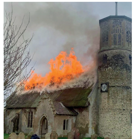
A spark from welding caused the blaze at St Mary's church in Beachamwell, Norfolk (Photo: Norfolk Churches Trust)
