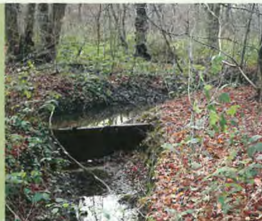
A sluice in Mad Bess Wood, Ruislip
