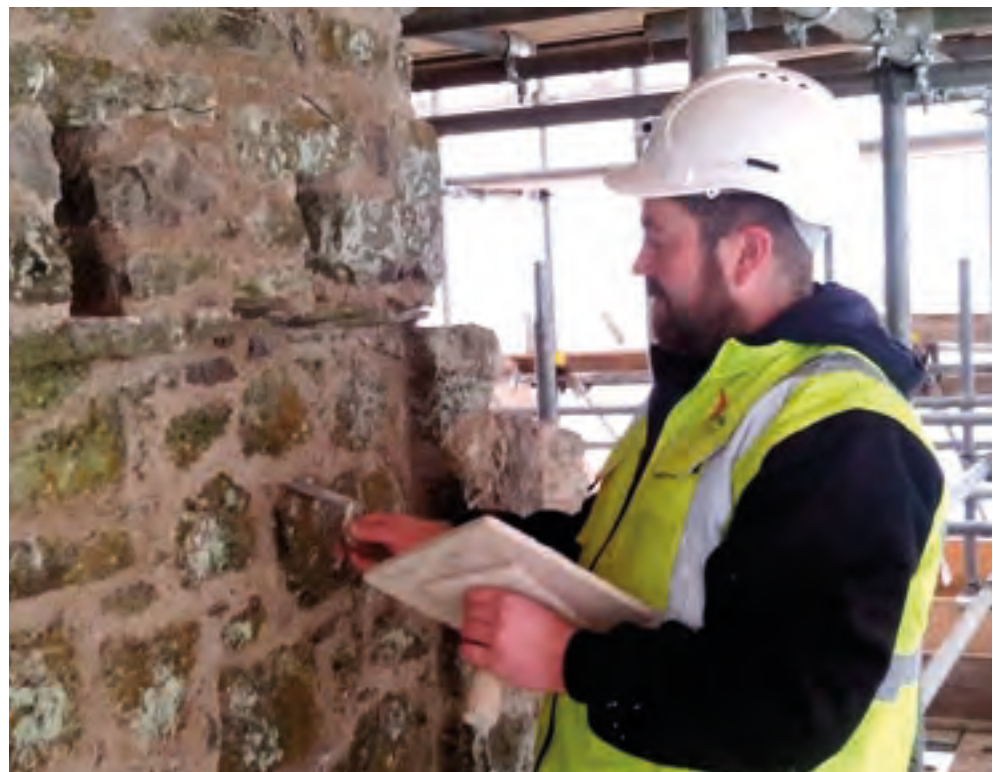
Conor O'Brien, apprentice stonecutter/stonemason working on conservation of the gate tower at Kells Priory, Co. Kilkenny
