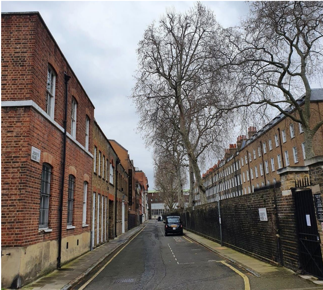
Figure 2.14: Jockey's Lane - former mews now in use as offices
