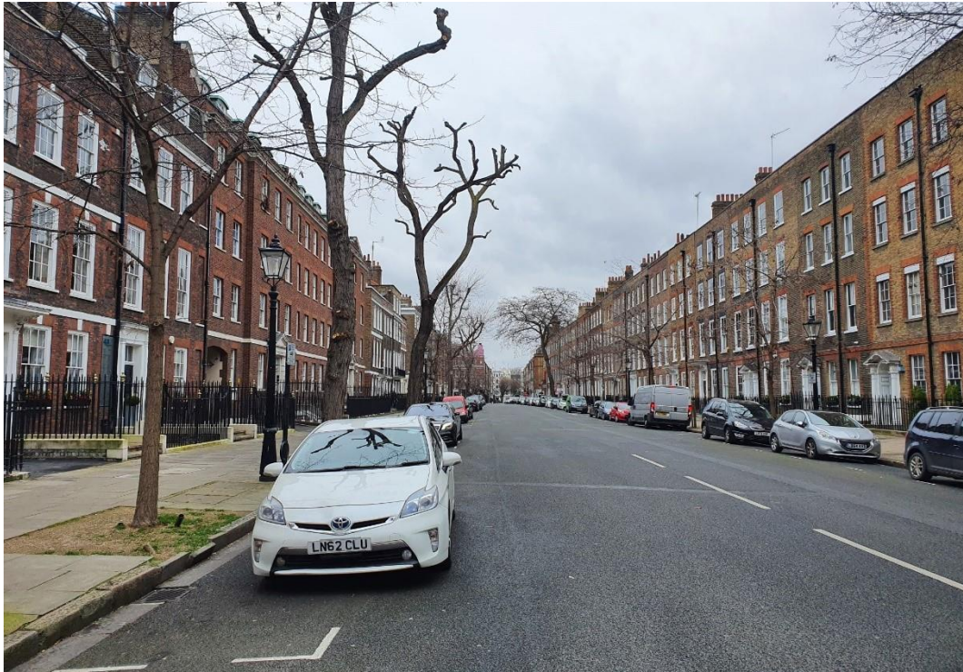
Figure 2.11: Buildings on Bedford Row looking north towards Theobalds Row
