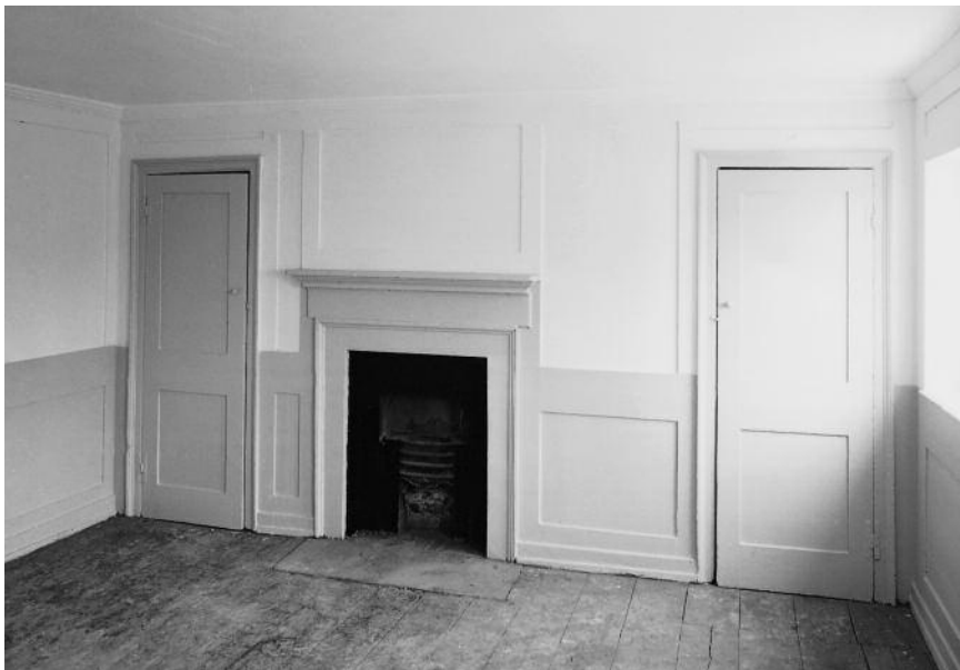
Fig. 5. The second-floor front room in No. 116 Deptford High Street in 1974. London Metropolitan Archives
