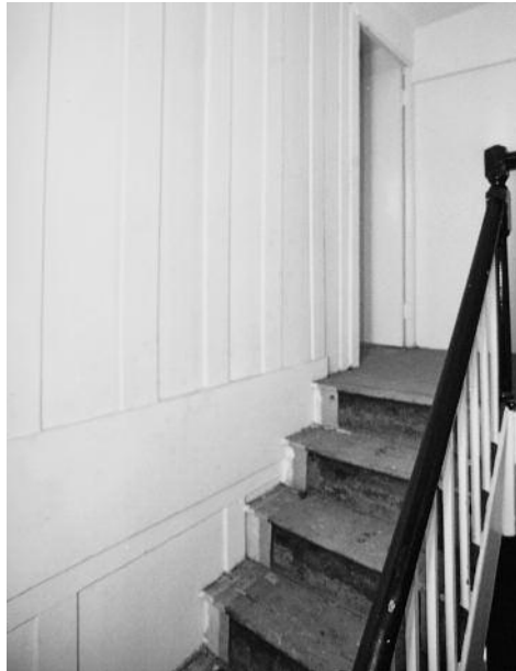
Fig. 6. The head of the staircase on the second floor in No. 106 Deptford High Street in 1998, showing the plank-and-muntin partition to the back room.
