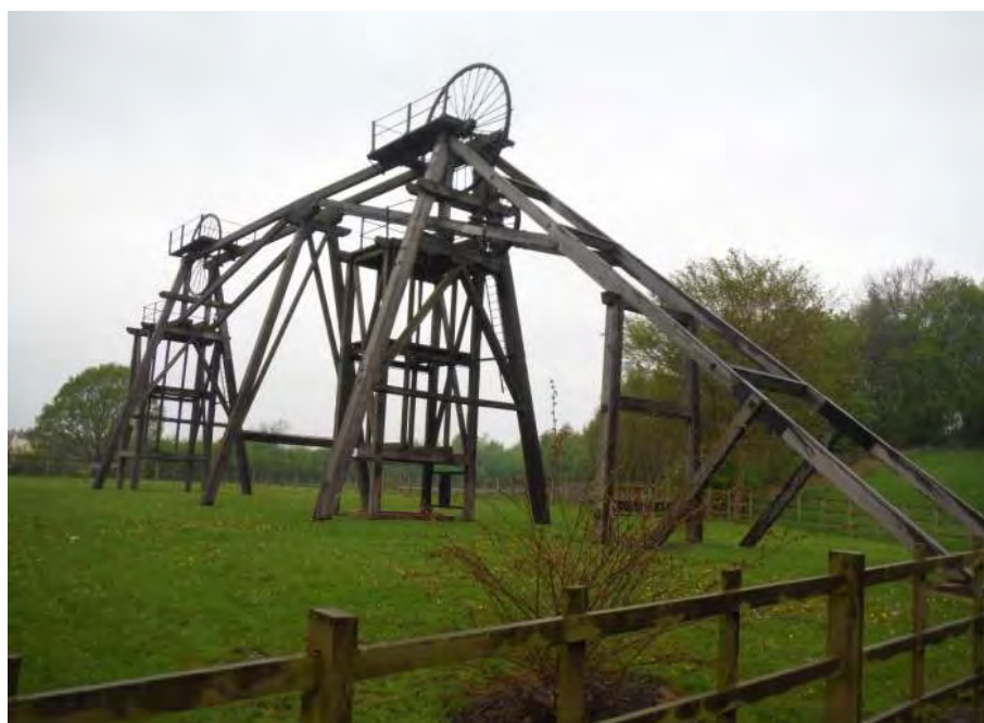
Plate 19: Brinsley Headstocks (Photograph DSCF9927)
