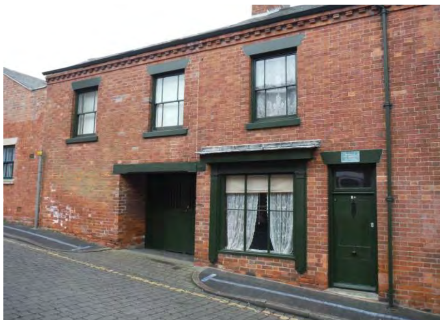
Plate 31: Victoria Street (Photograph DSCF9913)
