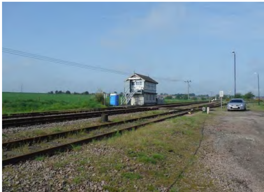
Plate 54: Mineral railway from Thoresby Junction (Photograph DSCF0736)
