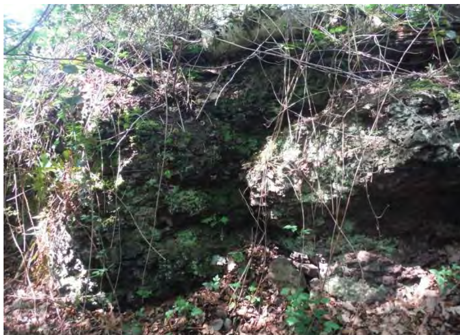
Plate 5: Old coal pit (5, 170), now wood, to the east of Babbington (Photograph DSCF0310)
