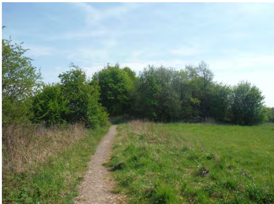
Plate 34: Embankment for the former mineral railway (looking south), now covered in vegetation (Photograph DCF9797)
