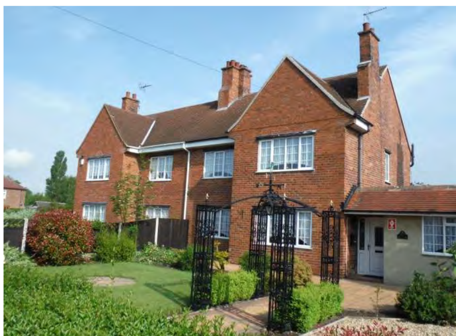
Plate 56: Houses to Ollerton Road (Photograph DSCF0759)
