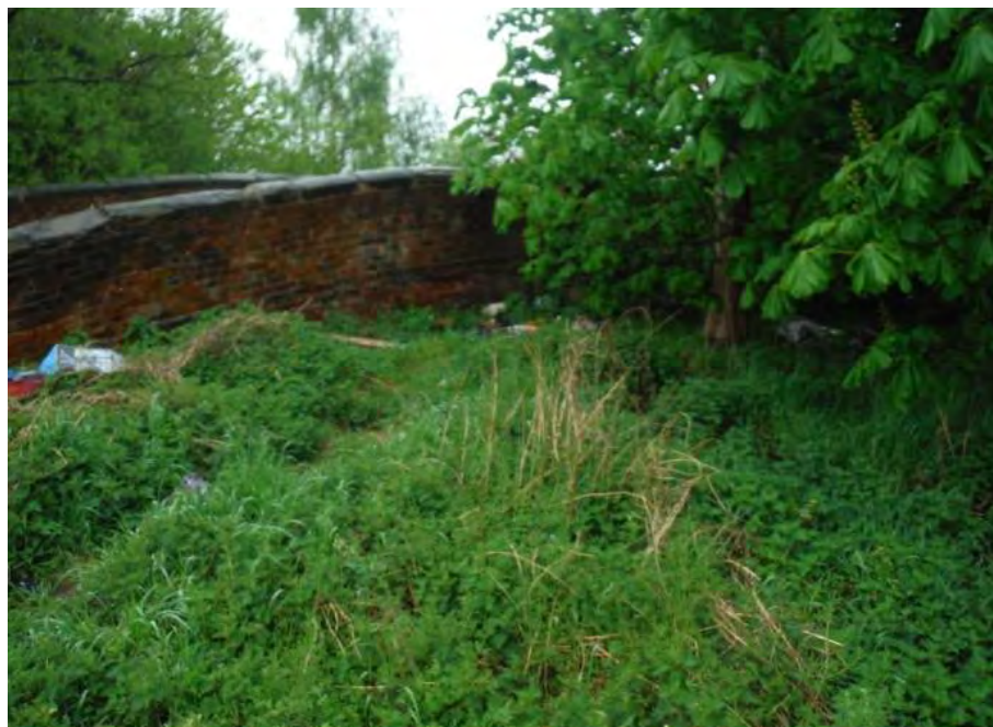
Plate 24: Overgrown section of the Nottingham Canal (Photograph DSCF9963)
