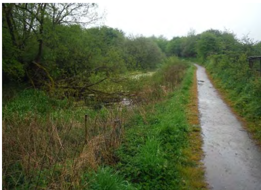
Plate 25: Overgrown section of the Nottingham Canal (Photograph DSCF9965)
