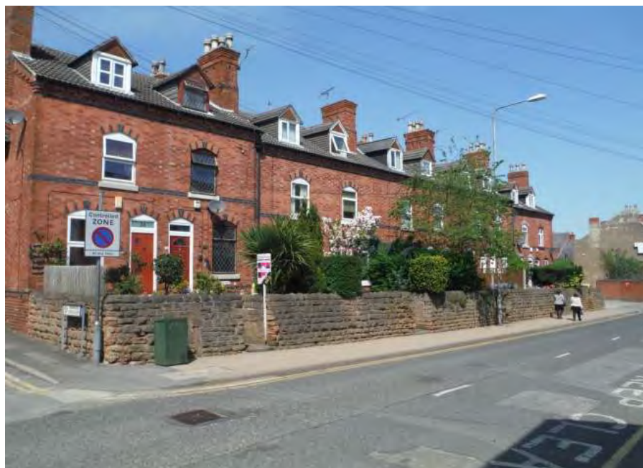
Plate 37: Deputies Row on Watnall Road in Hucknall (Photograph DSCF0029)
