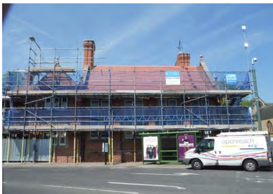
Plate 40: Hucknall Free Library under refurbishment (Photograph DSCF0009)
