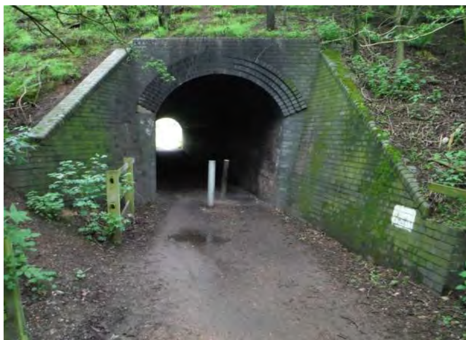
Plate 44: Photograph of bridge over former mineral railway (Photograph DSCF003)
