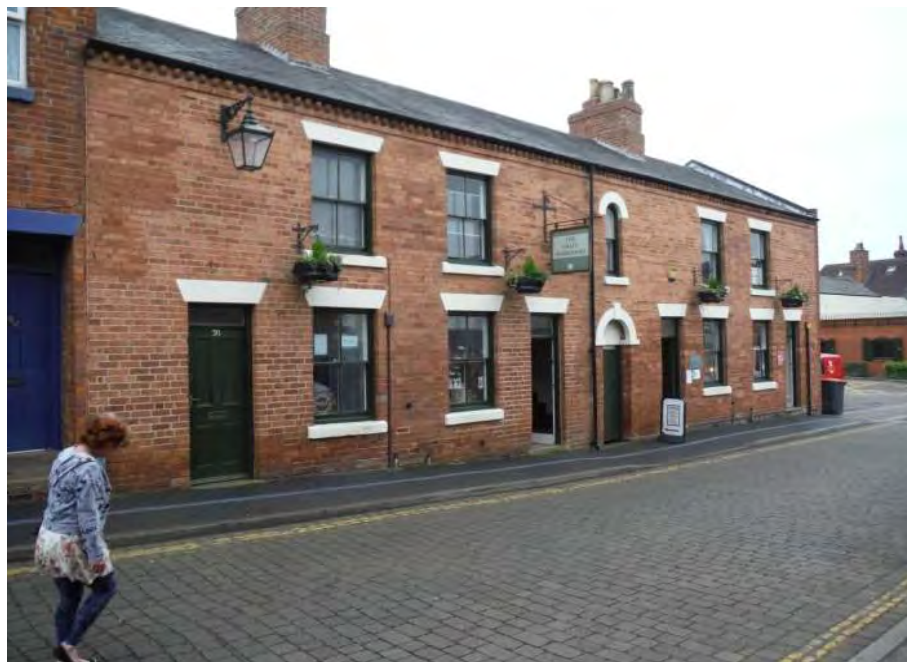
Plate 30: Houses on Scargill Walk, The Squares (Photograph DSCF9905)
