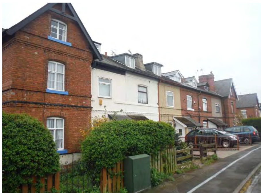
Plate 26: The Breach general view (Photograph DSCF9858)
