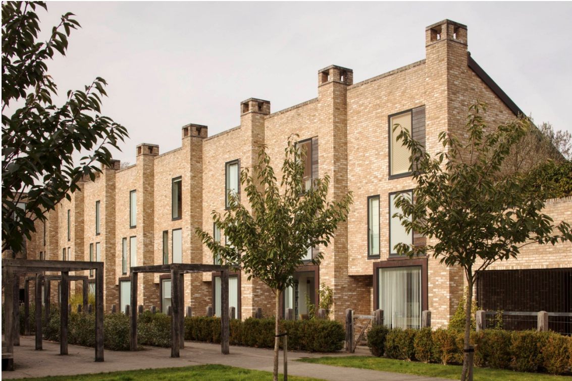
Modern high density terraced housing at Accordia. © Historic England Archive, Patricia Payne
