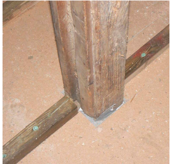
Figure 8: Insulation has been laid into the space between the floor joists. © Oxley Conservation
