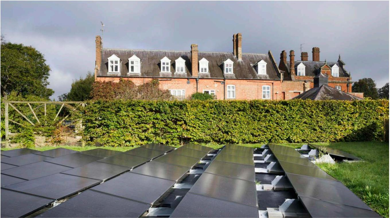
**Figure 12:** Ground mounted solar panels set behind a hedge at Chippenham Hall, Cambridgeshire.
