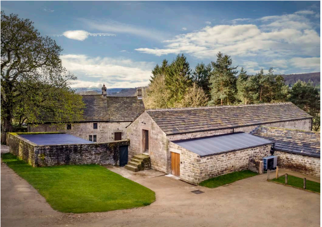
Figure 11: An air source heat pump has been installed in an inconspicuous location behind a barn next to the Grade II listed farmhouse.
