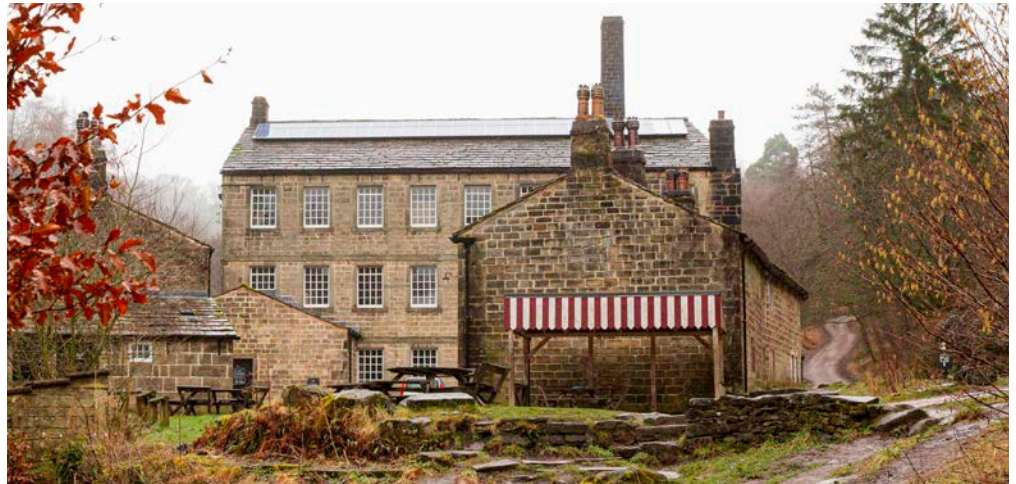
Figure 2: Photovoltaic panels were installed on the rear roof slope of the Grade II listed Gibson Mill (NHLE 1226169), West Yorkshire, a 19th-century cotton mill. © National Trust
