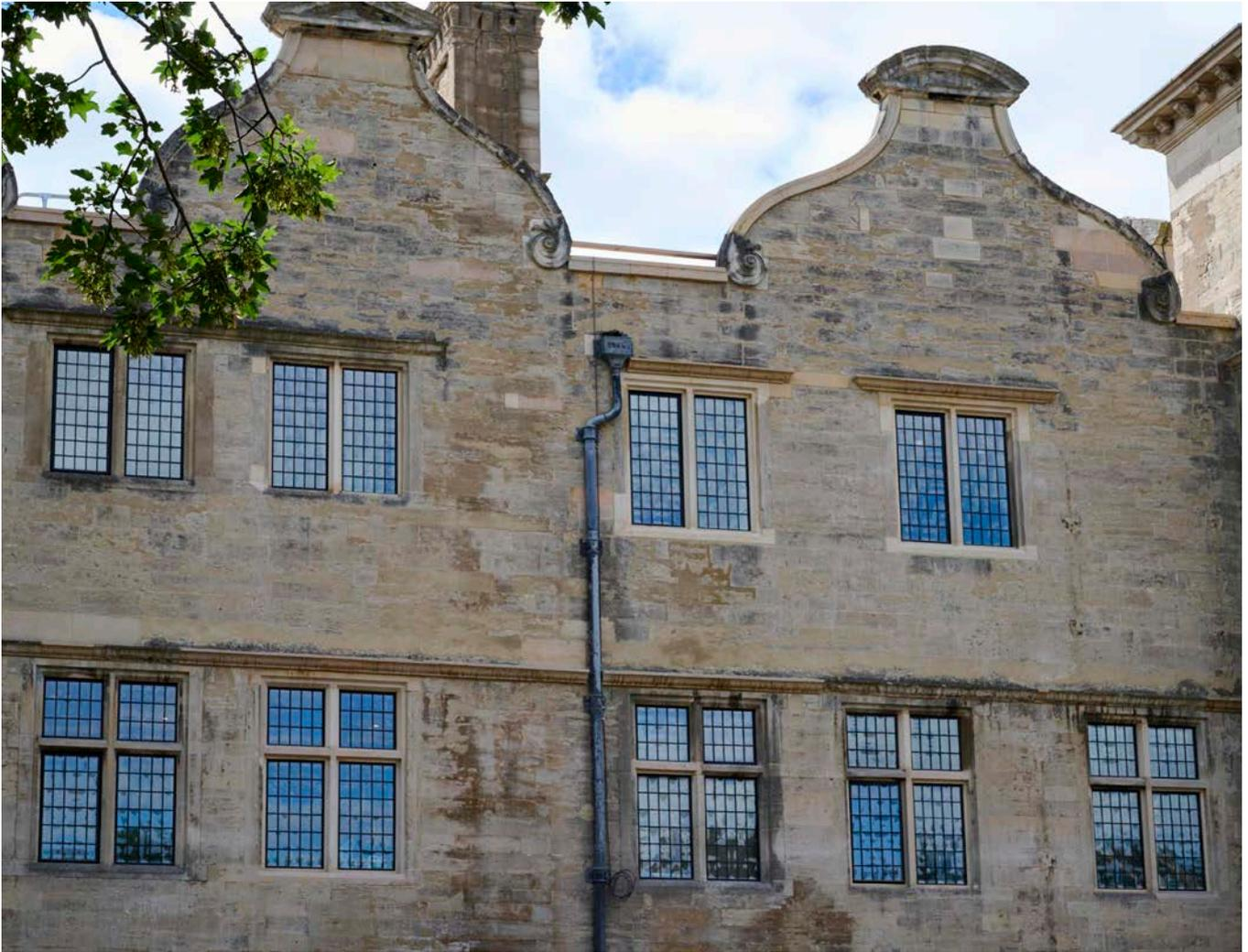
**Figure 4:** In this Grade I listed building, a number of existing metal-framed windows were replaced with either mono-laminated glass or slim-profile double glazing.
