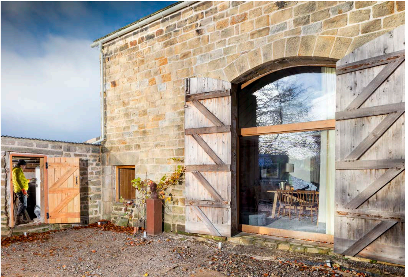
Figure 9: An exterior view of Hoggerstone Hill Farm, showing the converted barn and the outhouse containing the ground source heat pump. © Historic England
