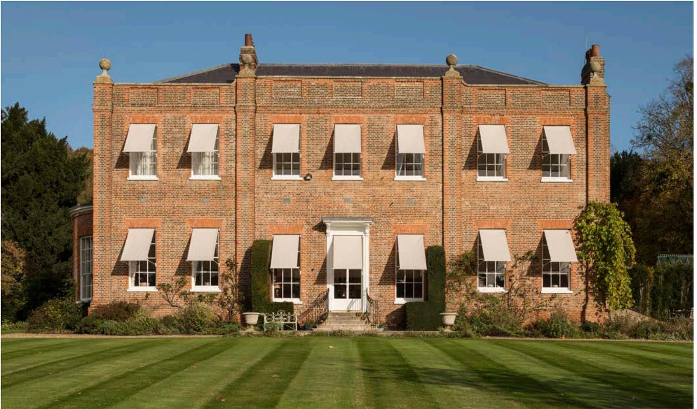
**Figure 14:** Rooms on the southwest elevation of this Grade II\* house increasingly suffered from overheating in summer. Historic fixings for external awnings were identified in the window reveals and replacement blinds were fitted.
