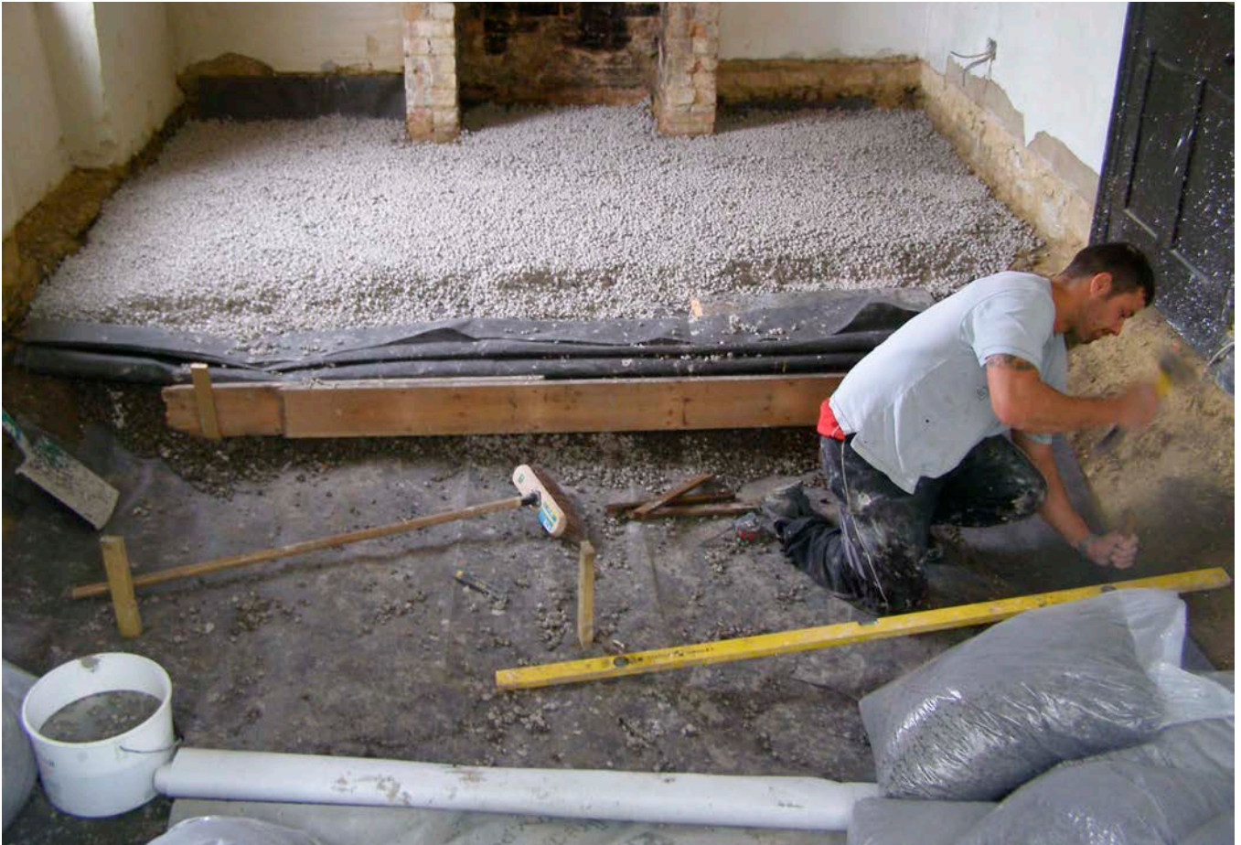
Figure 6: An insulated hydraulic lime floor being laid. © Matthew Clements/Mike Wye Ltd
