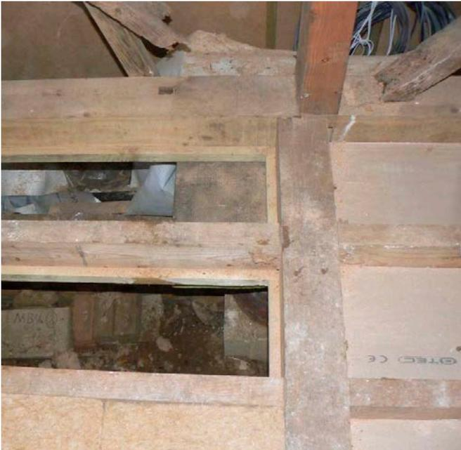
**Figure 7:** Battens have been added at the sides of the joists to support boarding to carry compressible sheep's wool insulation. © Oxley Conservation
