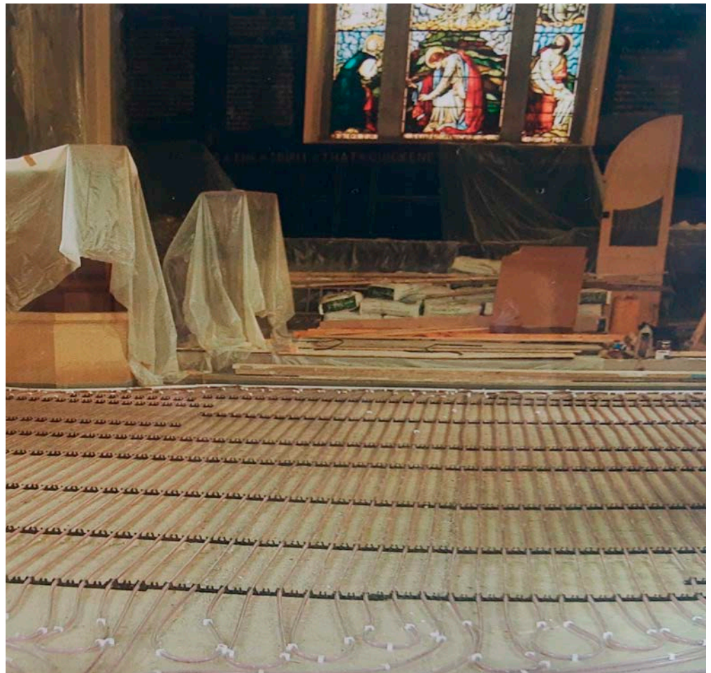
Figure 17: Site 4: Underfloor heating was laid during refurbishment works.
