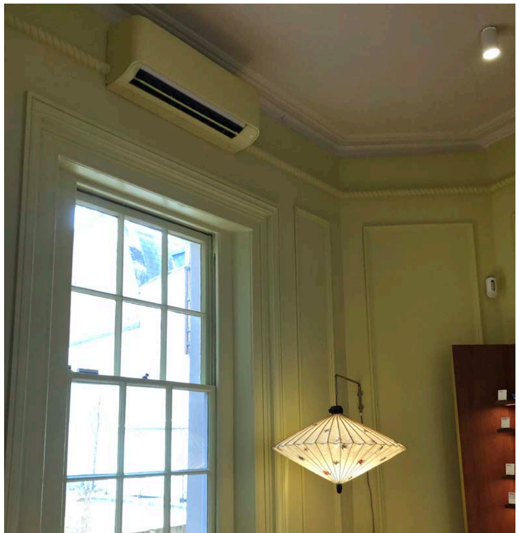
Figure 2: An example of a typical wall-mounted indoor condenser often used with DX ASHPs for both heating and cooling. The indoor condenser has been colour-matched to blend with the decor.
