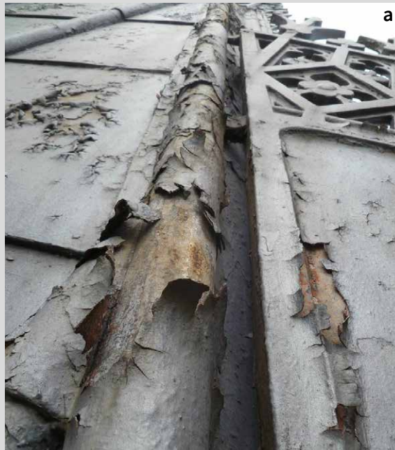
Palace of Westminster roofs project: (a) Cast-iron 'tiles' prior to repair
