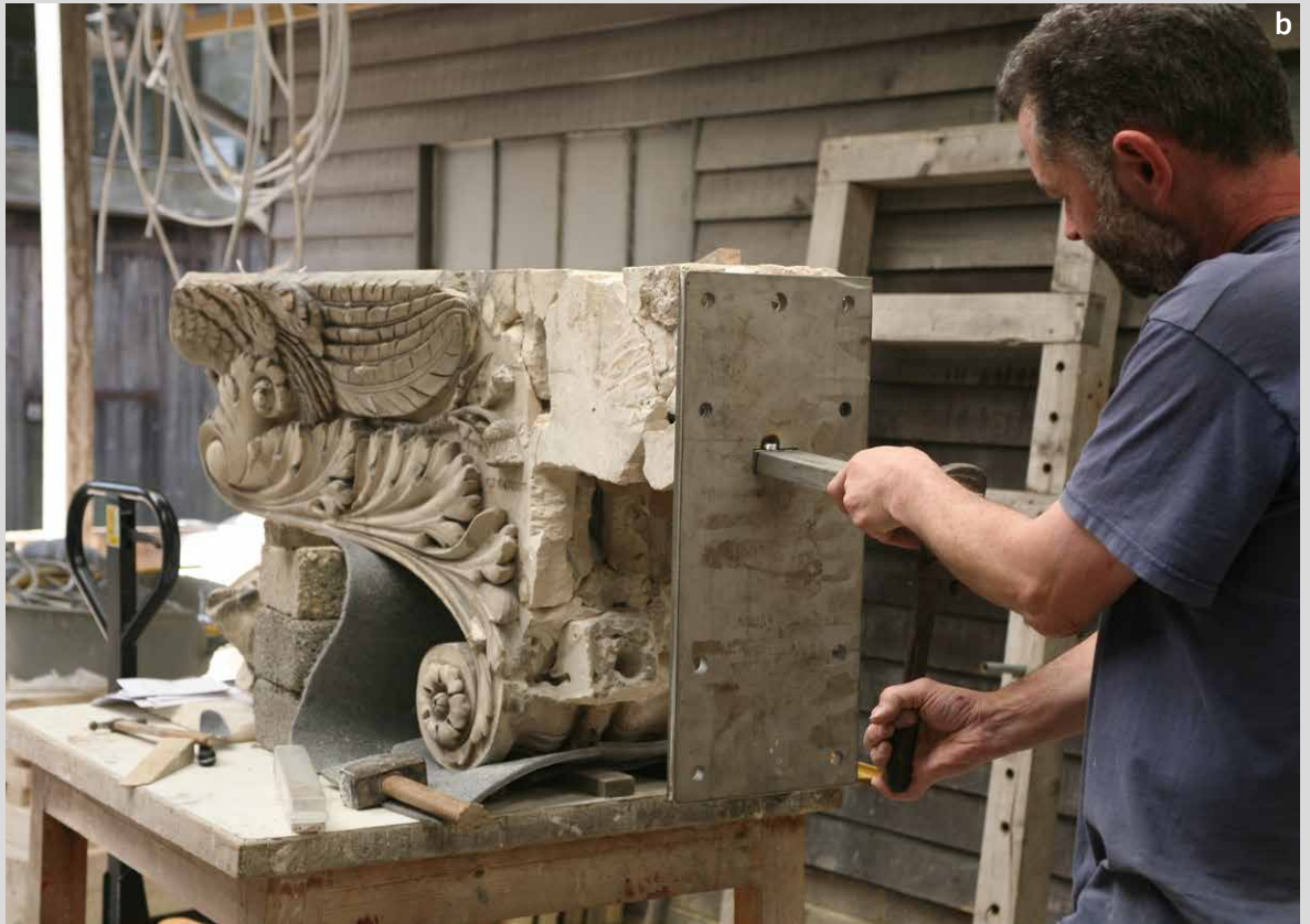
(b) Bracket being repaired in the workshop (c) Repaired bracket in situ
