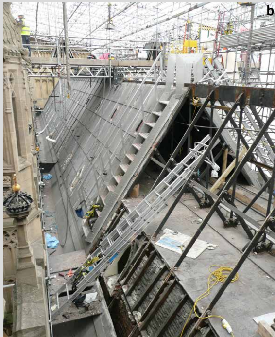
(b) Repair work in progress
