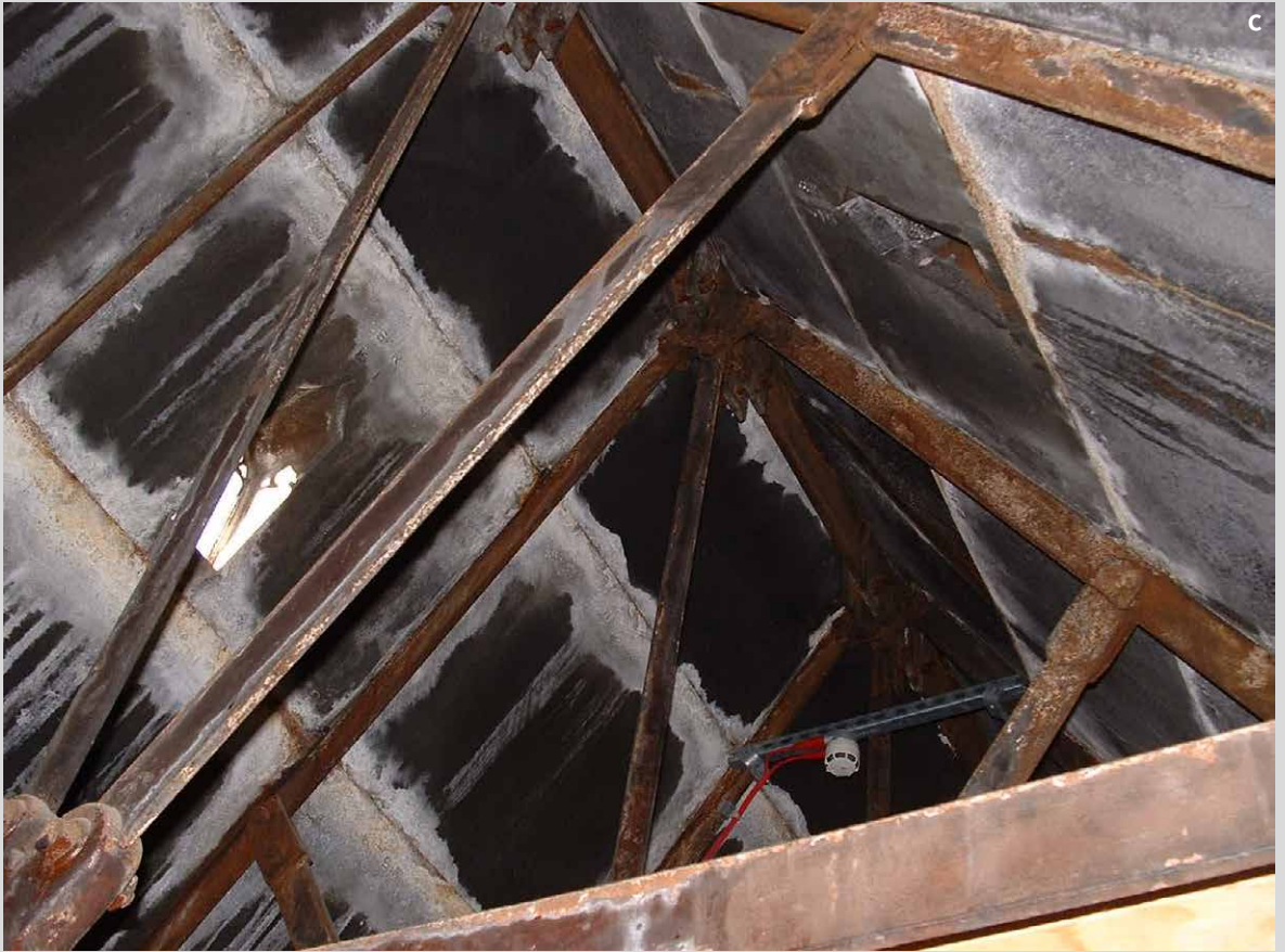
(c) Iron roof trusses
