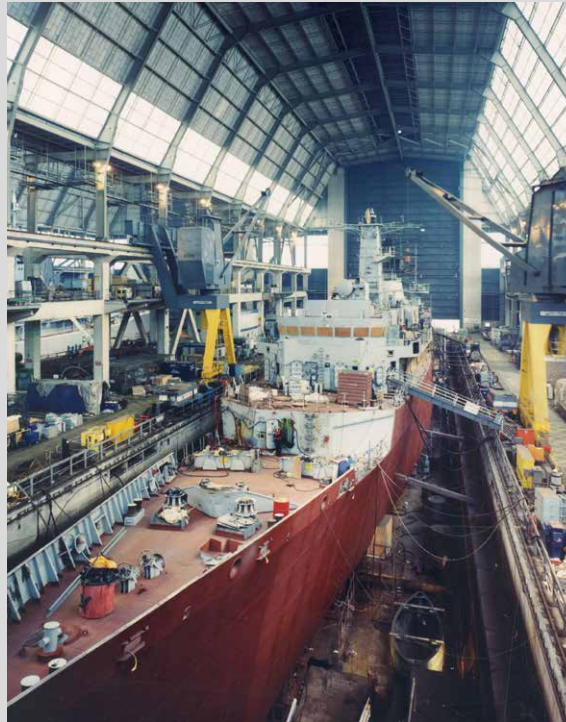
HM Naval Base Devonport: the Frigate Complex completed in 1977
