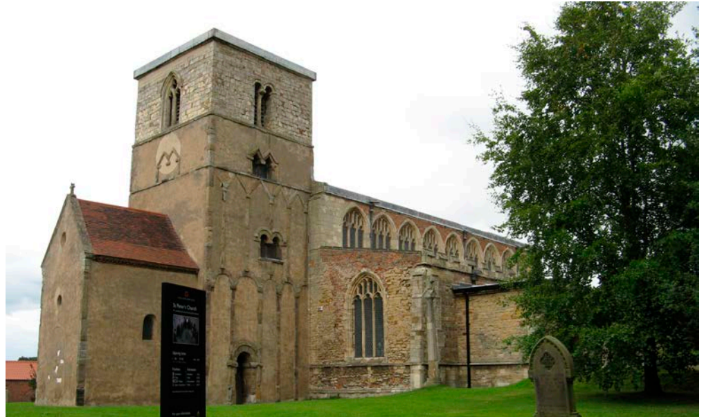
Figure 14: Church of St Peter, Barton-upon-Humber. Carboniferous Millstone Grit Sandstone.
