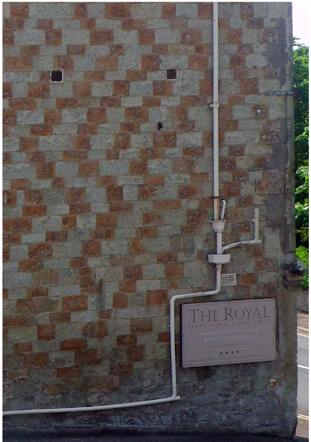
Figure 8: Royal Hotel annex, Ventnor. Ventnor Stone and Ventnor Foxstone.
