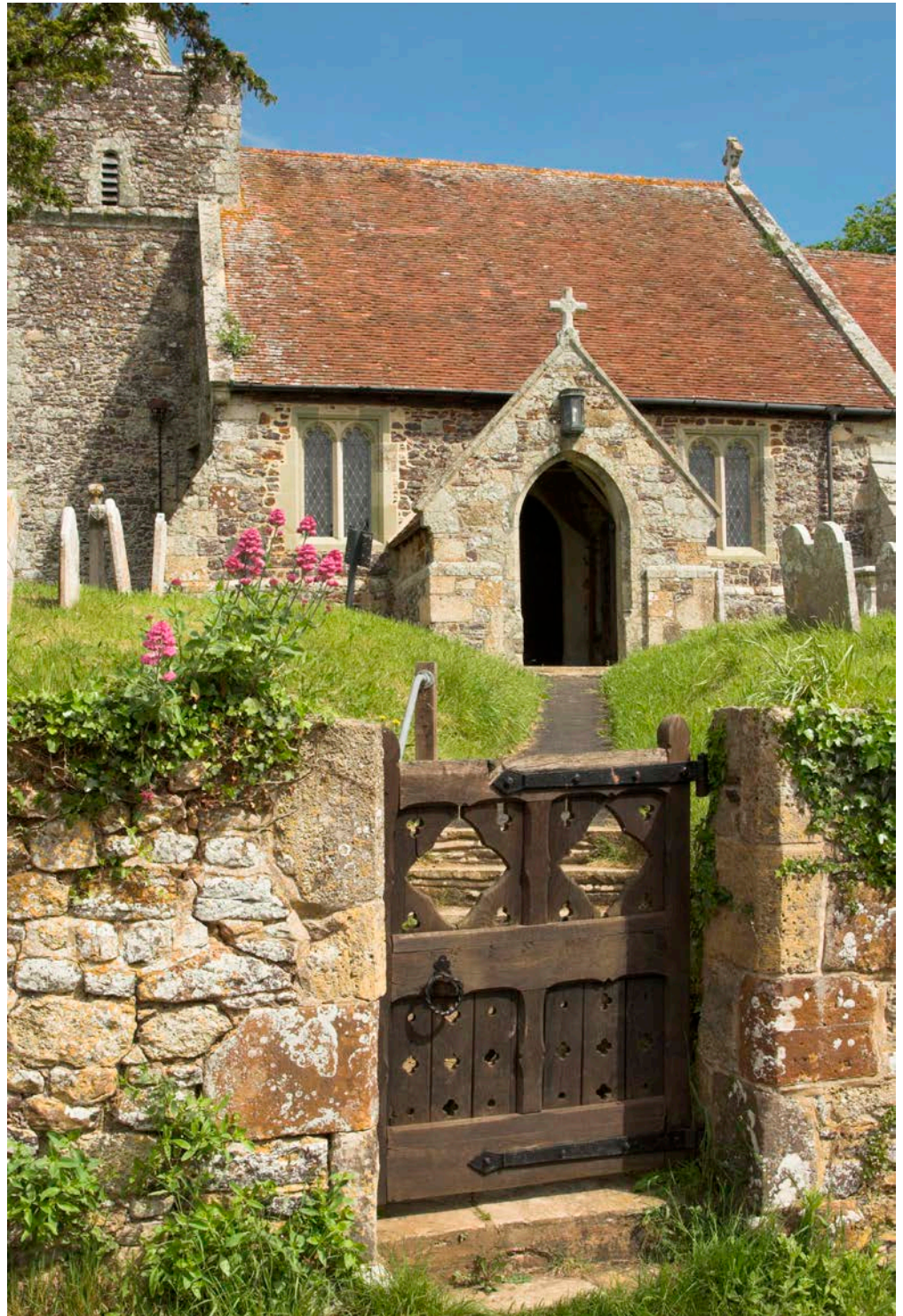
Figure 5: St Peter and St Paul's Church, Mottistone. Monk's Bay Sandstone and Upper Greensand Sandstone.
