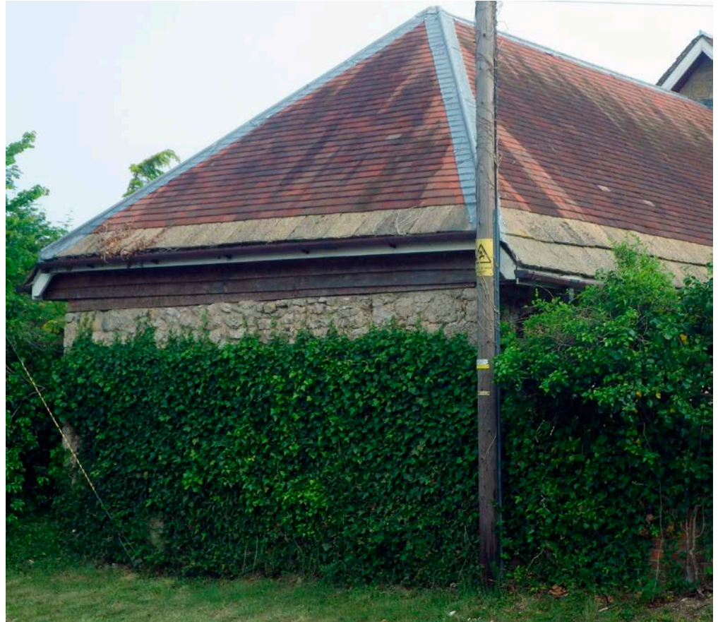
Figure 18: Farm buildings, Endfield Farm, Ningwood. Bembridge Limestone slate roofs.
