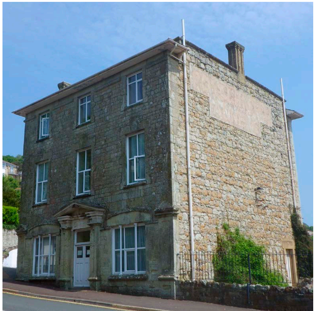
Figure 7: Royal Hotel annex, Ventnor. Ventnor Stone and Ventnor Foxstone.
