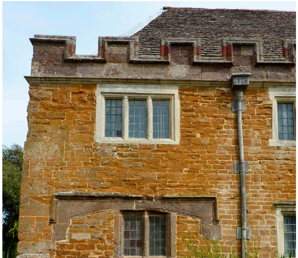
Figure 40: Nevill Holt Preparatory School, Nevill Holt. Northampton Sand decorative lintels and parapet.
