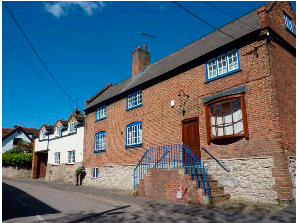
Figure 32: Houses, Grimes Gate, Diseworth. Diseworth Sandstone footings and garden walls.
