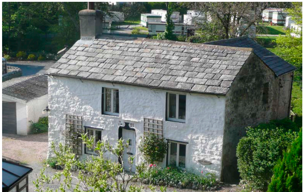
Figure 11: Cottage, Ingleton. Ingleton Slate roof.
