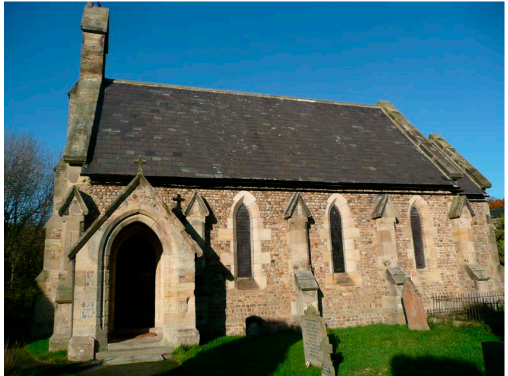
Figure 43: Church of St John the Evangelist, Mickley. Fluvial/fluvio-glacial material from the River Ure with Welsh purple Penrhyn Slate roof.
