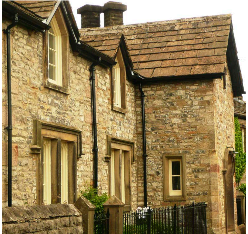
Figure 16: Redberry House, Broughton. Broughton Limestone and Millstone Grit sandstone quoins, window dressings and roof slate.
