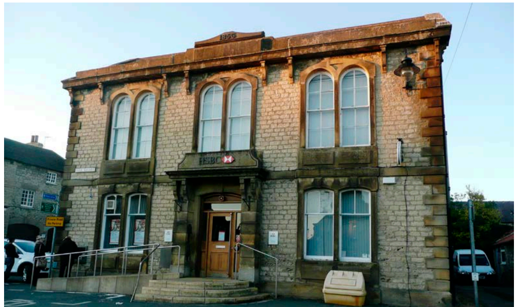
Figure 41: 14 Park Square, Masham. Cadeby Formation limestone with ashlar sandstone dressings.
