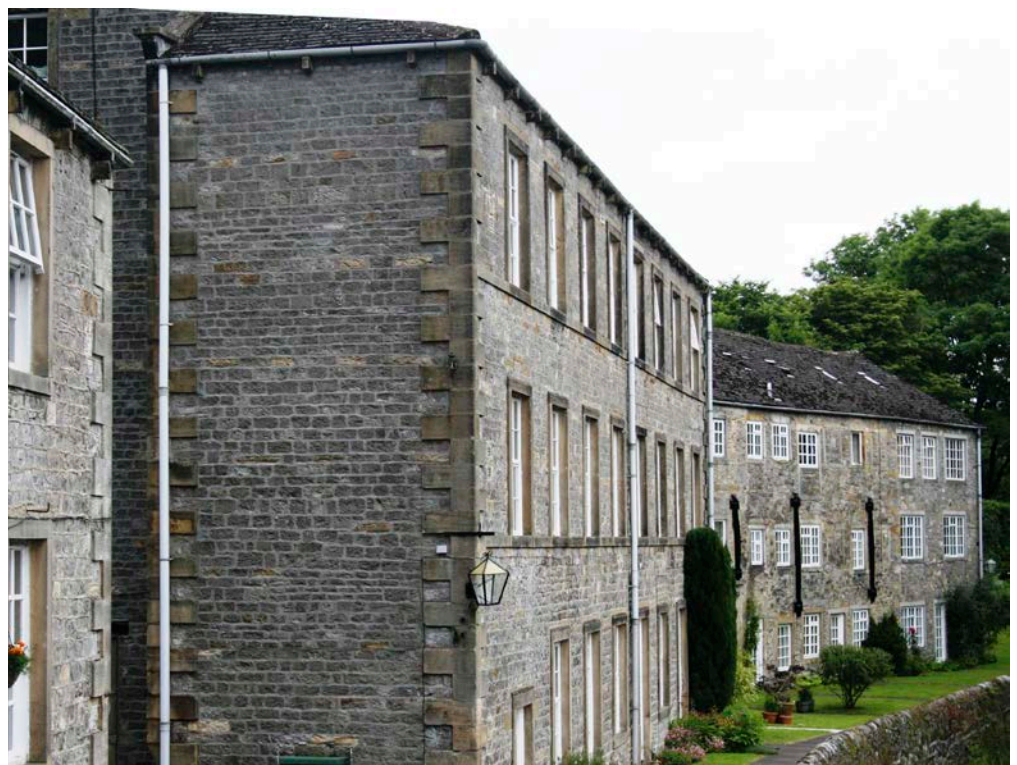
Figure 15: Airton Mill. Thornton Limestone facing and Millstone Grit sandstone quoins and window dressings.
