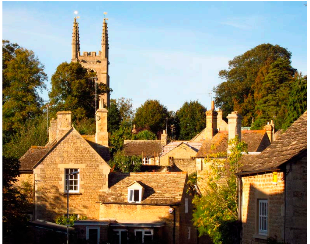
Figure 16: Houses, Easton-on-the-Hill. Lower Lincolnshire Limestone, Collyweston Stone slate roofs, with Ketton Stone quoins and window frames.
