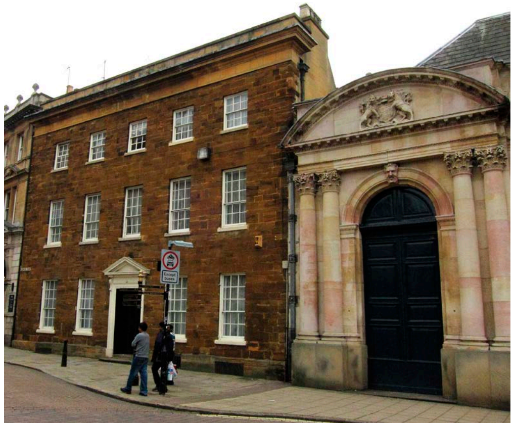
Figure 9: Left, The Judge's Lodgings, George Row, Northampton. Northampton Sandstone facade. Right, Sessions House, Northampton. Ketton Stone.
