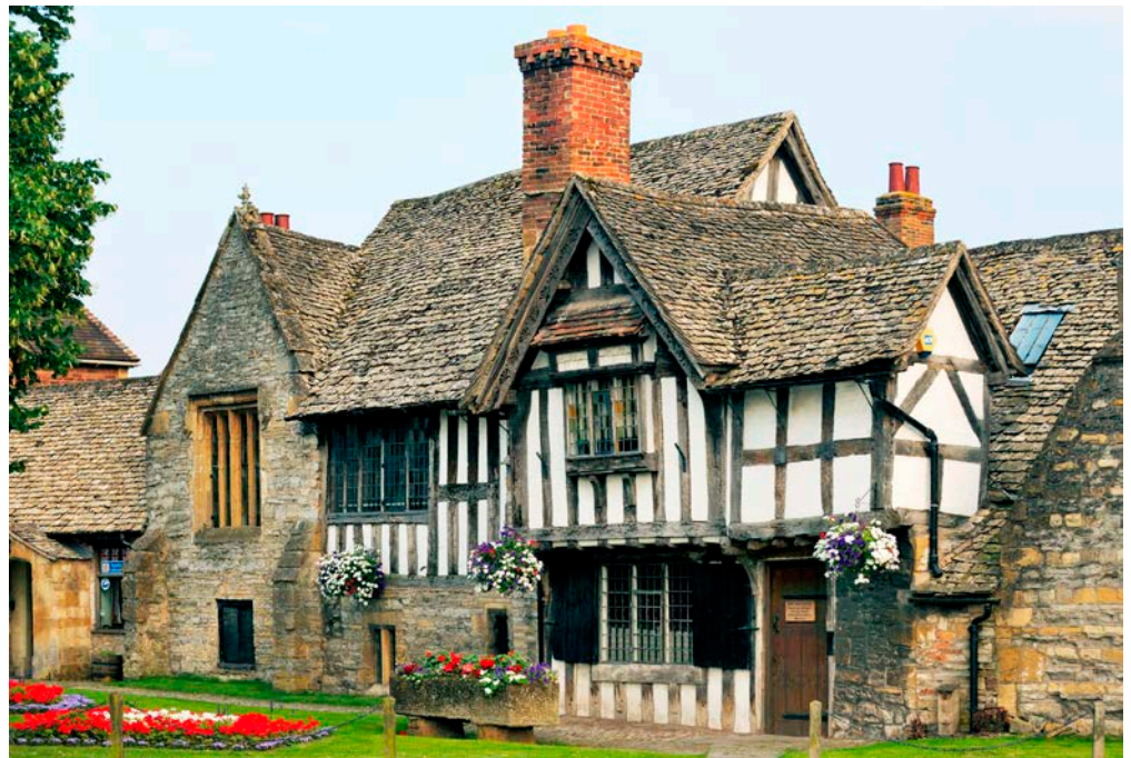
Figure 25: The Almonry, Evesham. Blue Lias and Cotswold limestones, Cotswold slate roof.
