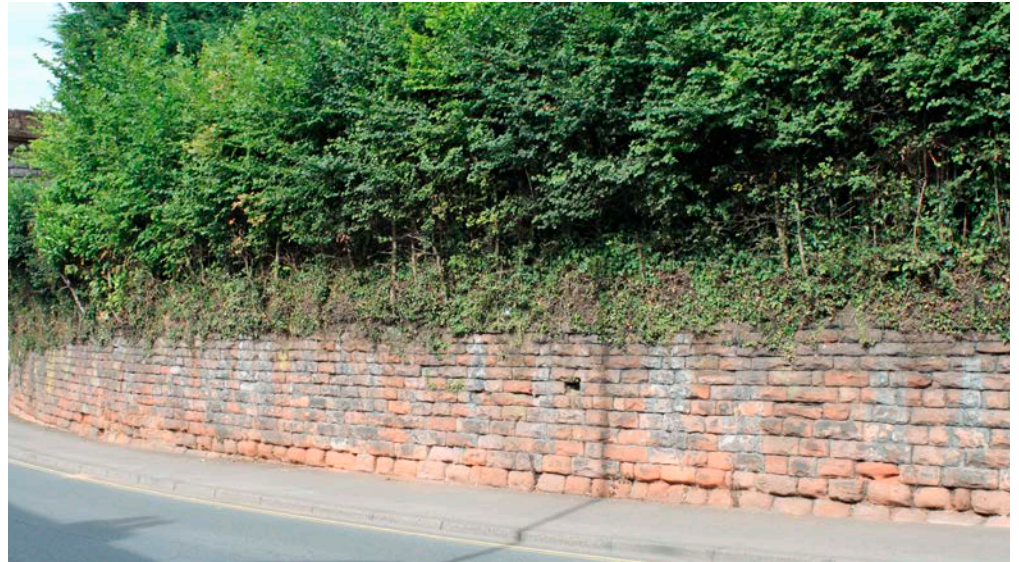
Figure 17: Wall, Bewdley. Bridgnorth Sandstone.
