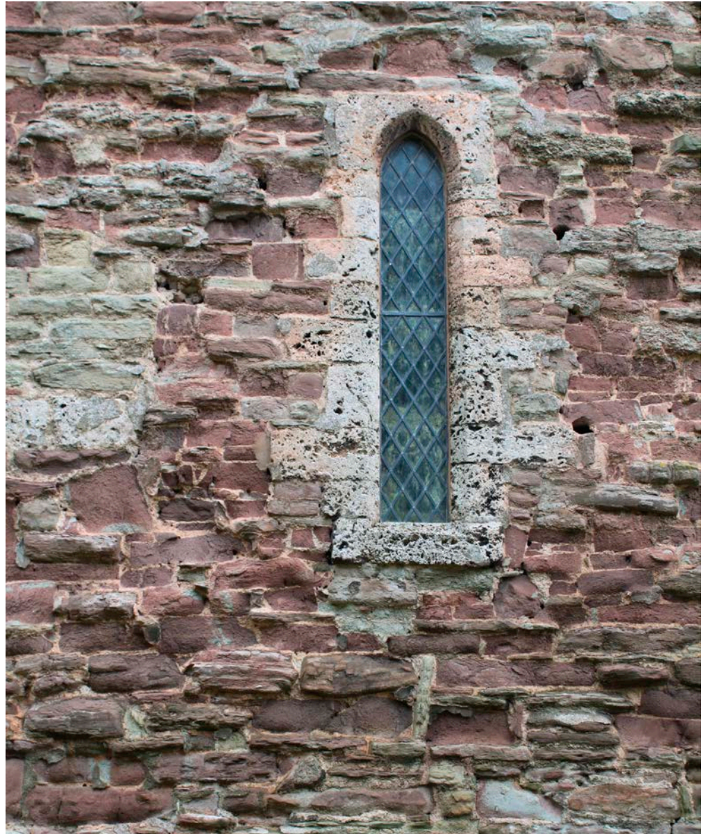
Figure 7: St Kenelm's Church, Clifton on Teme. St Maughans Formation sandstones. Tufa window surrounds.
