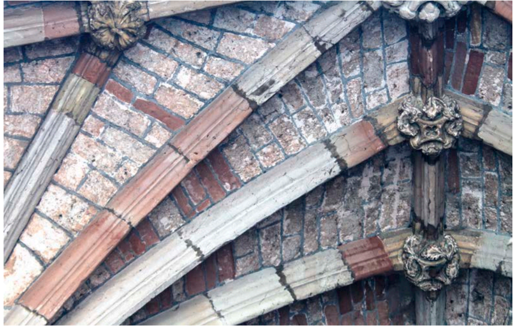
Figure 28: Worcester Cathedral. Tufa between the ribs.
