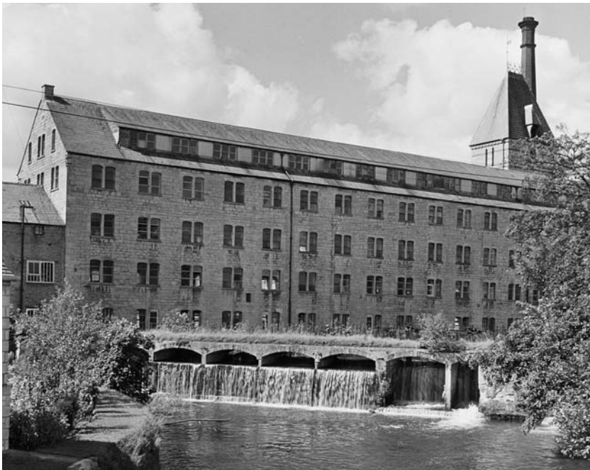
Ebley Mill, Stroud, Gloucestershire, as photographed by Eric de Mare in 1956 – one of more than a million NMR records now available online. Once one of the largest woollen-cloth mills in Stroud, the building is now the headquarters of Stroud District Council.
