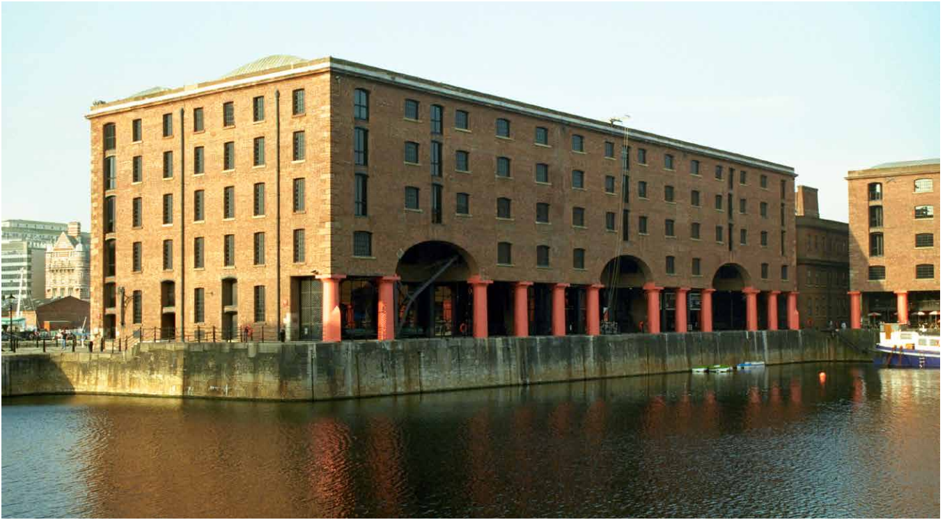
Figure 4 Warehouse D in Liverpool's Albert Dock (listed Grade I). An iron-framed building by J Hartley of 1841-5, standing five storeys high.
