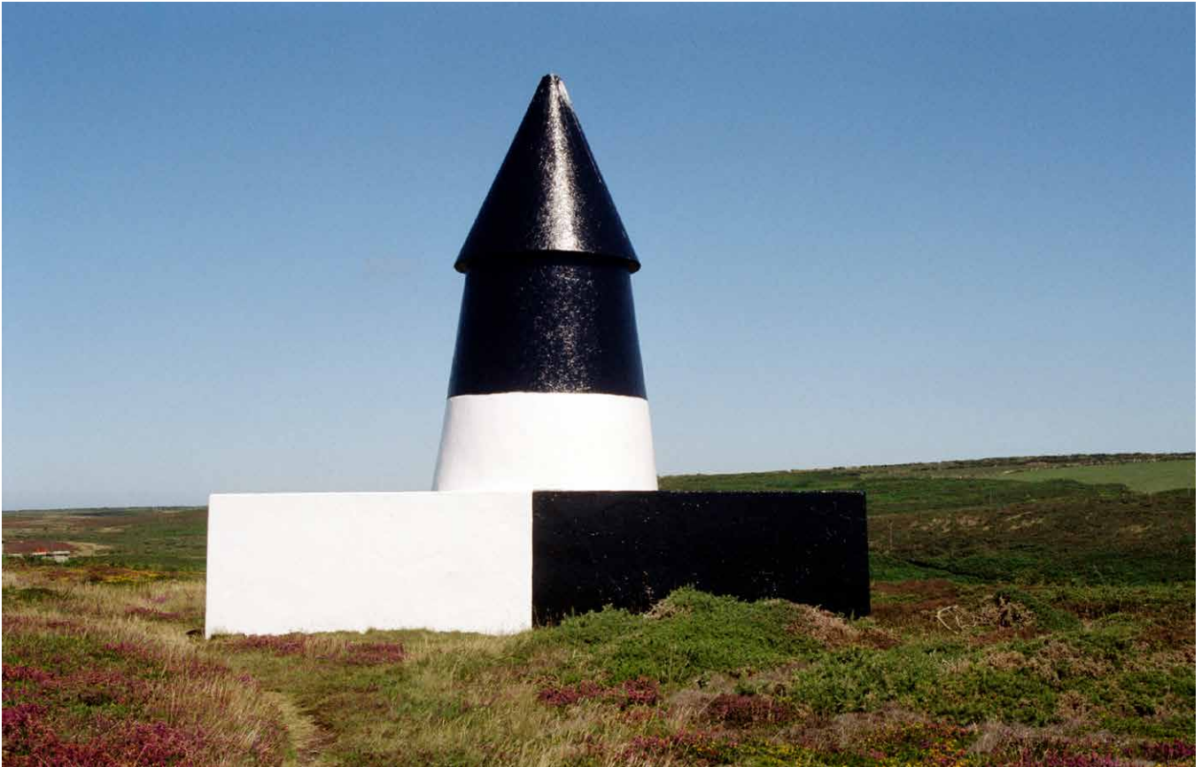
Figure 8 The daymark at St Levan, Porthgwarra, Cornwall (listed Grade II). This was erected in 1821 to mark an alignment with the Runnel Stone Reef.
