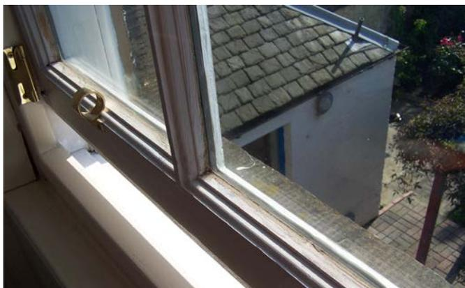
Left: The original timber window frame can accommodate new double-glazing, making the change visually discreet.
