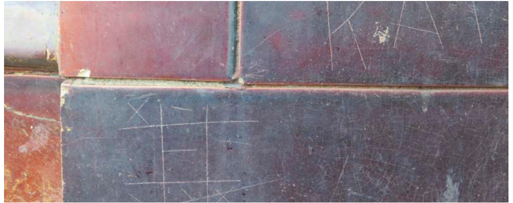
Figure 23: Graffiti has been scratched into the smooth glassy surface of faience (glazed terracotta) facing blocks. Located at the entrance to a historic pub, these marks include a game of noughts and crosses and are typical of casual vandalism.
