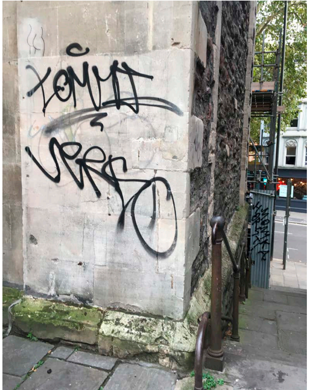
Figure 18: Repeated graffiti incidents and cleaning attempts on this Portland limestone masonry have resulted in an unsightly appearance. Faded remains of past graffiti are visible on the lighter, previously cleaned area, which contrasts in colour with the uncleaned masonry above.
