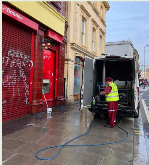
Figure 41: Mobile graffiti removal equipment normally consists of a pressure washer, with component parts, hoses, compressor and water tank, all contained within a service vehicle. Water run-off from cleaning is typically directed into surface water drains. Consequently, chemical cleaners containing toxic environmental contaminants should not be used in mobile cleaning operations, unless waste water can be contained and disposed of separately.
