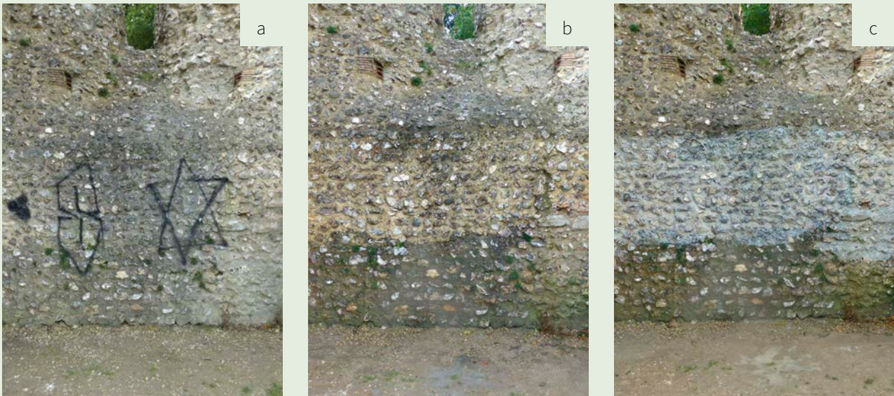
Figure 51: Internal walls of the Great Tower, Ludgershall Castle, Wiltshire (13th century), a scheduled ancient monument. a) Graffiti before removal. b) The wall after graffiti removal. c) The wall after application of a wax graffiti barrier. Masonry was allowed to partially dry before applying the coating. The wax remained opaque until it fully dried. When a wax coating is added to a wet or damp surface, a permanent 'bloom' can result. This can only be eliminated by removal of the wax.
