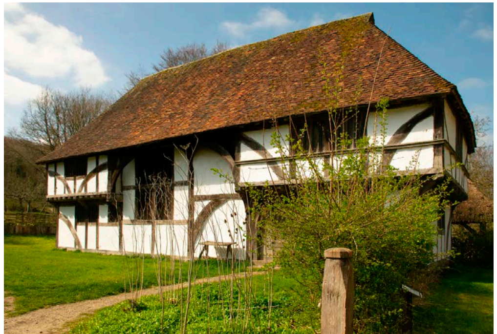
Figure 2: Bayleaf Farmhouse, a timber-framed Wealden hall house originally from Chiddingstone in Kent, re-erected at the Weald and Downland Museum in Singleton, West Sussex. © Andy Bliss
