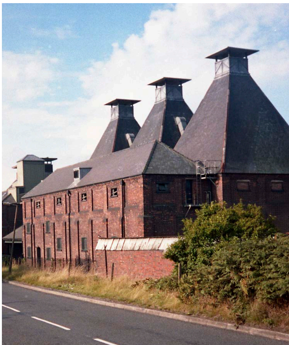
Above: Wolverhampton and Dudley Brewery Maltings, Langley Green, Oldbury: exterior with pyramidal roofed kilns. The maltings was designed by Arthur Kinder in 1898. © Amber Patrick
