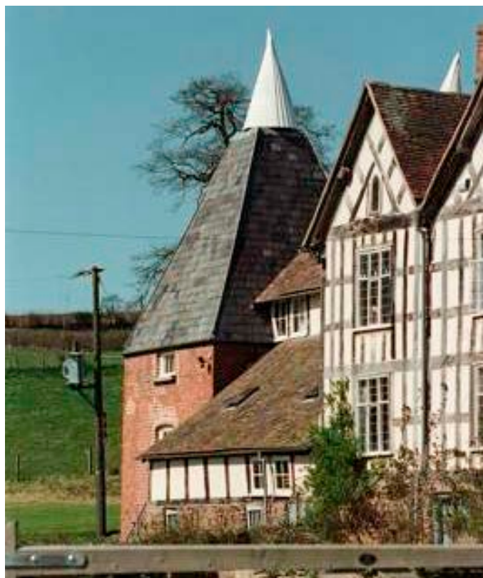
Above: Lower Venn, Avebury, Herefordshire. Note the kiln directly attached to the farm house. 2003. © HE IOE1/09397/07
