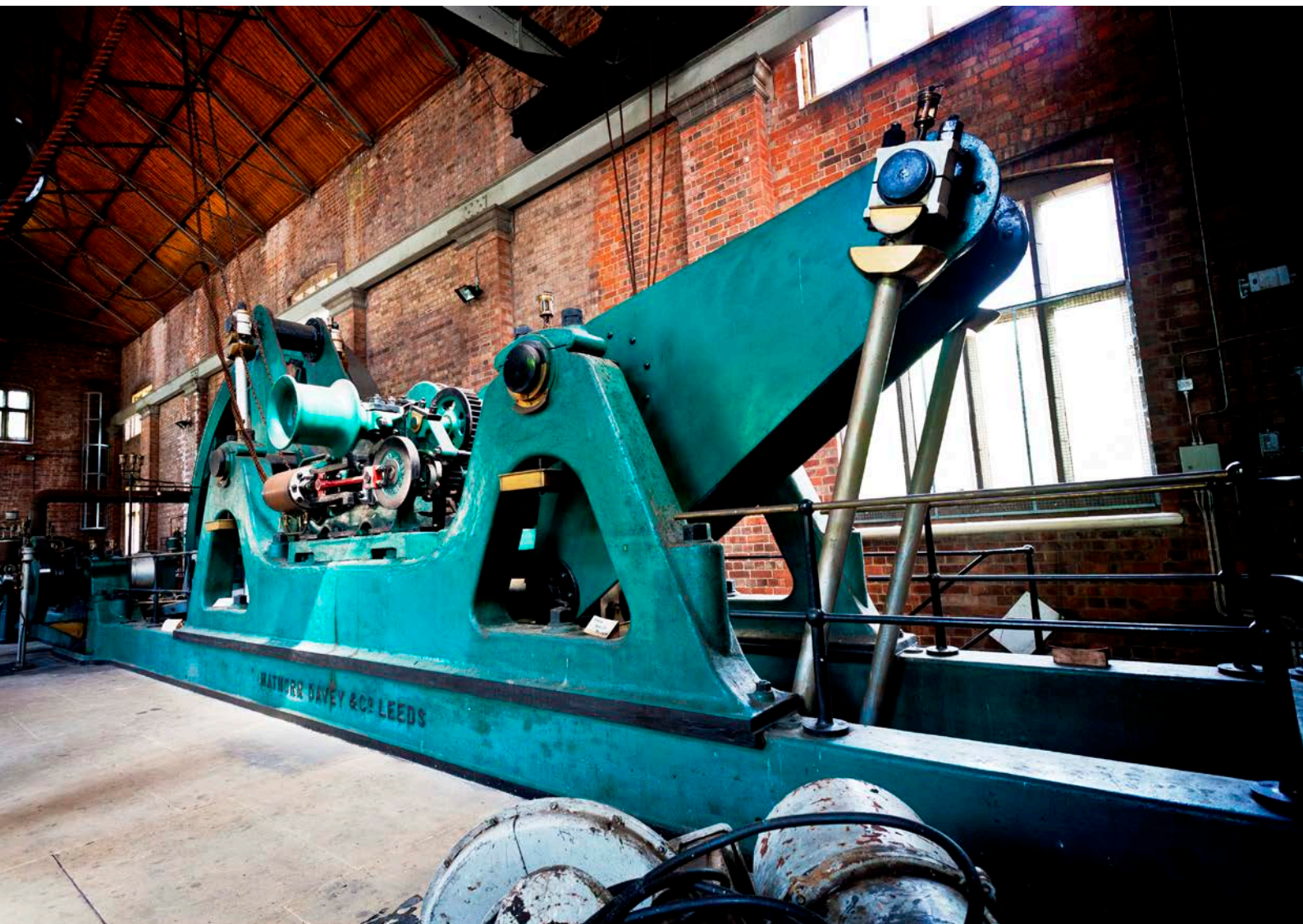
Above: The conserved horizontal steam engine at Brindley Bank waterworks (1903) in Staffordshire. © Morturn, Public Domain
