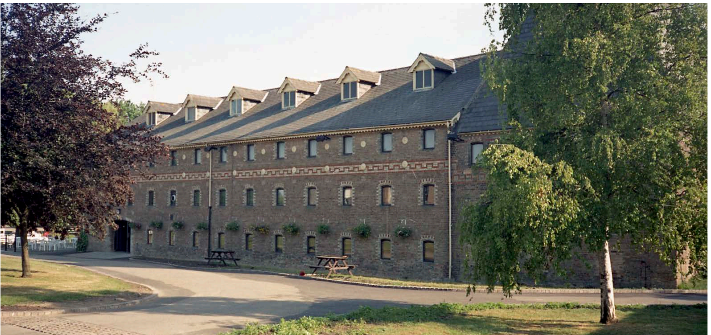
Above: The Maltings Theatre, Ship Lane, Ely. The kiln survives but is hidden by the tree on the right hand side. © Amber Patrick
