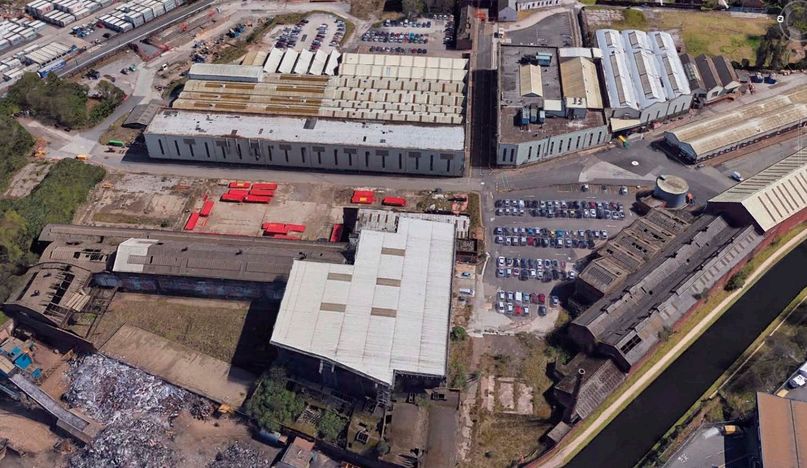
Above: 3-D oblique aerial photo of the Soho Foundry looking east. The protective roof was erected over the main Foundry building in 2006. Courtesy of Google Earth 2020
