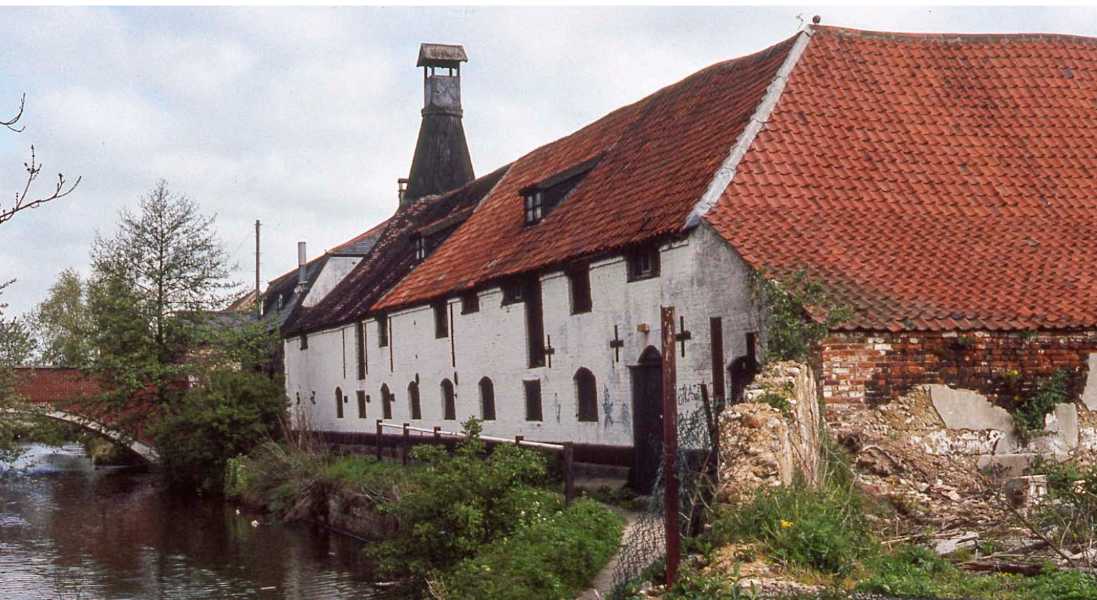
Above: Malthouse between Prentice Road and Station Road, Stowmarket: the kiln is away from the camera and small windows face onto the Navigation. © Amber Patrick
