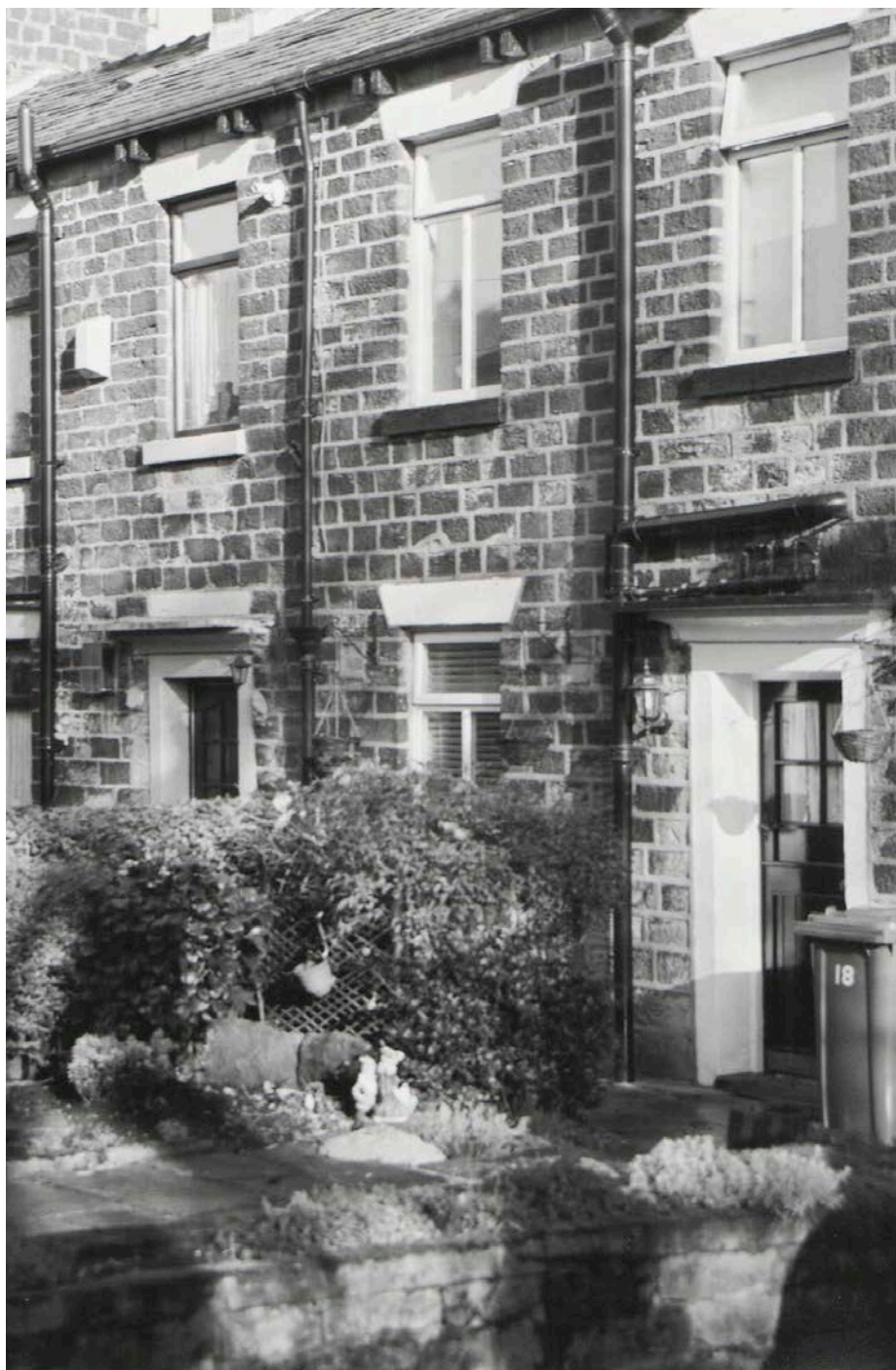
Above: Part of one of the three-roomed back-to-back house rows at Barrow Bridge. © Geoff Timmins
