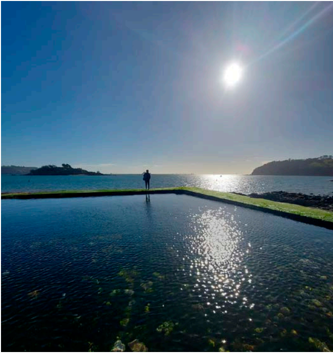
Above: Firestone Bay tidal pool, built about 1935, catalogue No. 12. © Joseph Panes, 2023
