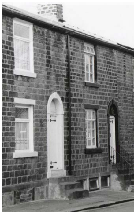
Above: Former handloom weavers' cottages, West View Place, Blackburn. A row of windows, now blocked, was provided in the cellars, along with a light well in front of them. © Geoff Timmins
