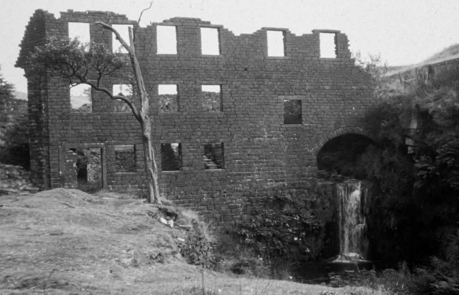
Above: Cheesden Lumb Mill, near Rochdale, a water-powered cotton spinning mill. The site made use of a natural fall of water.
