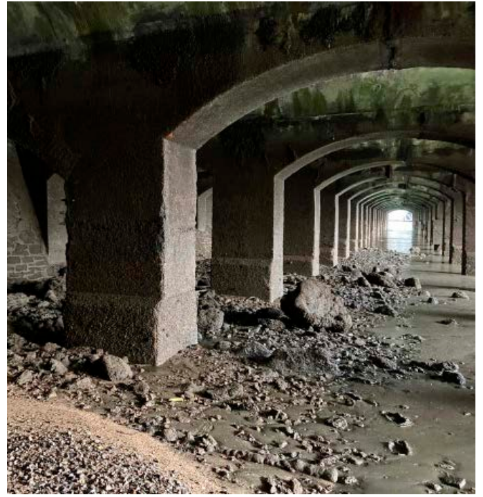
Above: Foundations of Trinity Pier, Millbay Docks 1852 – 70, catalogue No. 20. © Joseph Panes
