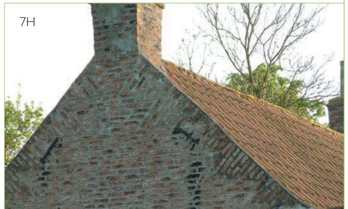
brickwork, which protects the cut brick of gable tops from the weather; a feature found from northern East Anglia to Northumberland, and the use of dentilled or cogged eaves.
