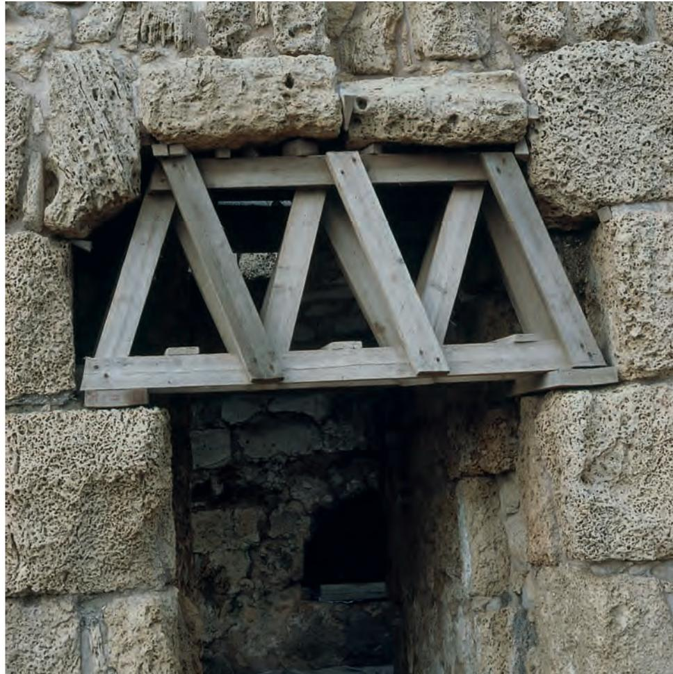
Decayed or missing jambs, lintels or mullions may require temporary support, either to allow further investigation or as part of the repair process. This is best done with timber struts or pins supported on either side of the opening.
