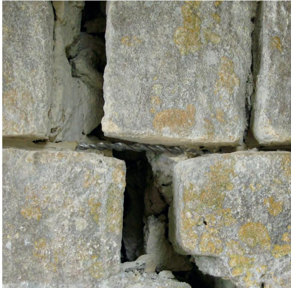
The diameter of the dowels will depend on the particular application, but can often be minimised by careful choice of location and direction. Helical ties, as their name suggests, are engineered uniform spiral dowels (usually galvanised steel or stainless steel) that, when fixed with grout or resin into a pre-drilled aperture, provide a strong, even anchorage into the masonry. They are available in various lengths and diameters.
