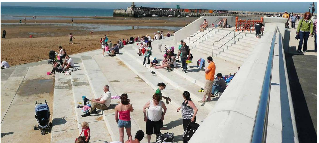
As part of its scheme to improve Margate seafront's resilience to coastal flooding and create new public realm, Thanet District Council constructed a stepped structure from the beach to the promenade. This innovative solution not only avoided the need for a high sea wall, but simultaneously created an excellent public space from which to enjoy views of the beach, sea and Stone Pier. The Steps have won numerous awards, including the national 2015 Civic Voice Design Award for Public Realm.
