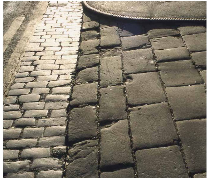
In Bideford, Devon, a ribbon of York stone paving flanked by cobbles provides a surface that is both traditional and accessible.
