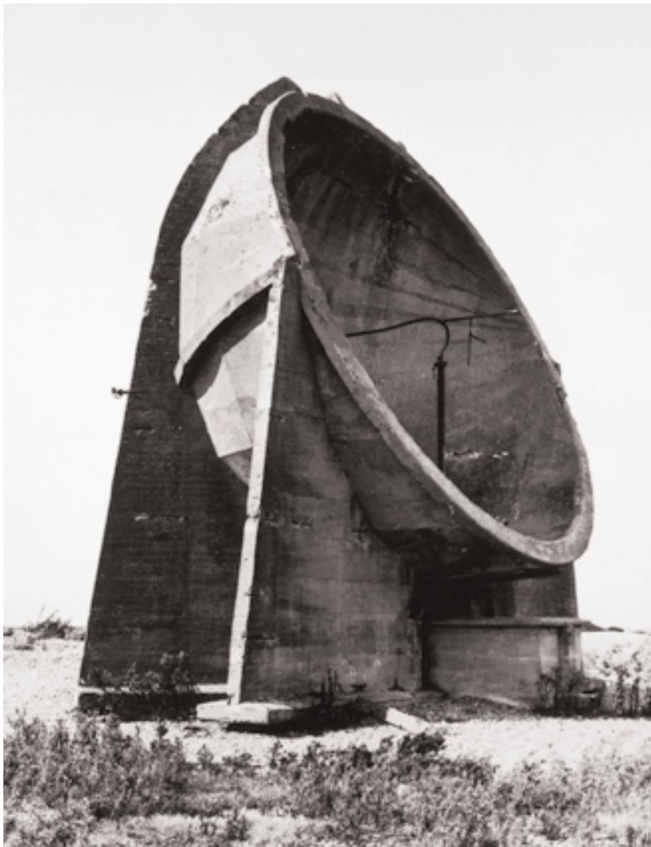
Early experiments in acoustic early warning systems resulted in the construction of concrete sound mirrors from 1917. This is part of a group at Denge in Kent, now a scheduled monument, which includes a 200ft (61m) strip mirror constructed between 1928 and 1930.
