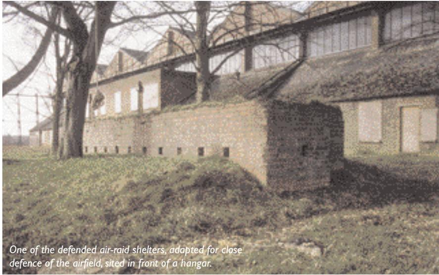
One of the defended air-raid shelters, adapted for close defence of the airfield, sited in front of a hangar.
