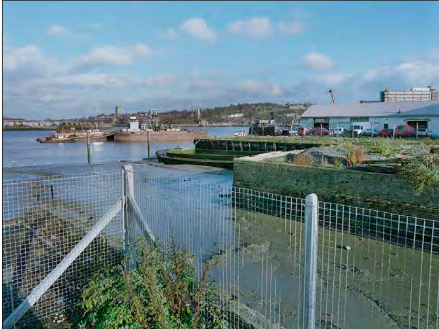
Fig. 99 Slipway to north of Gills Cottages photographed in 1995 [© Crown Copyright. Historic England Archive, AA95/06588]
