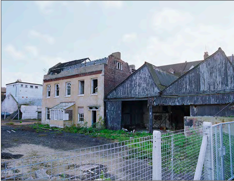
Fig. 20 Doust House and the remnants of the ship yard to the rear of No. 321 High Street Rochester photographed in 1995 [© Crown copyright. Historic England Archive, AA95/06585]
