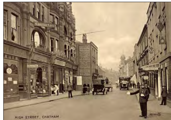
Fig. 24 Projecting premises on High Street Chatham in c.1925 indicating the previous building line [Medway Archives, DE402-15-41(L)]
