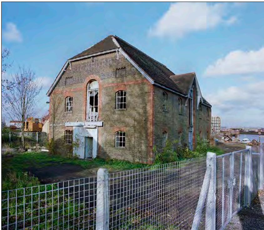
Fig. 94 Sheldrake House before restoration, photographed in 1995 [© Crown Copyright. Historic England Archive, AA 95/06590]
