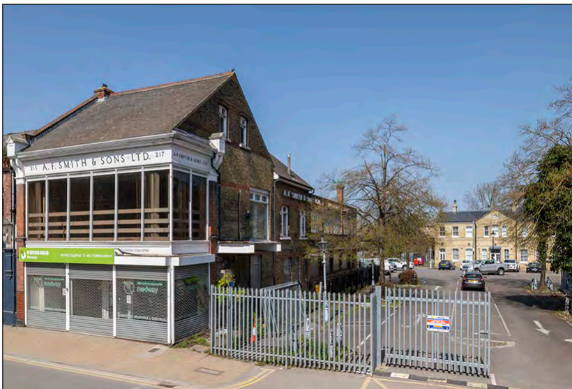
Fig. 95 The former Rochester Railway Station set back behind its forecourt [Chris Redgrave ©Historic England Archive, DP289294]
