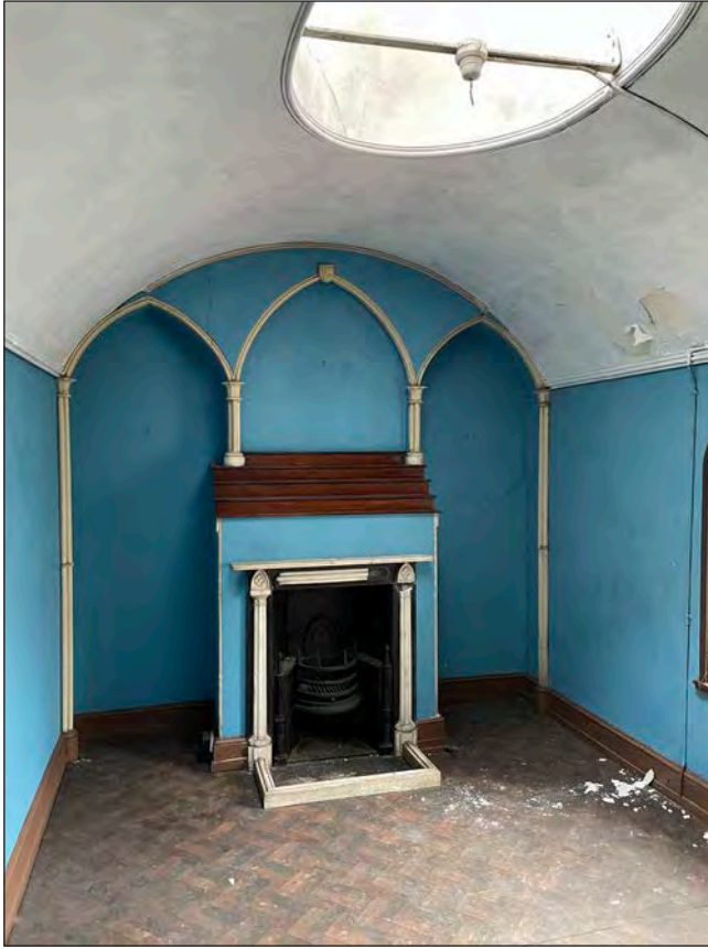
Fig. 68 The 'chapel', first floor, north-east wing view from the south [Posy Metz ©Historic England HSLSE09/P4]
