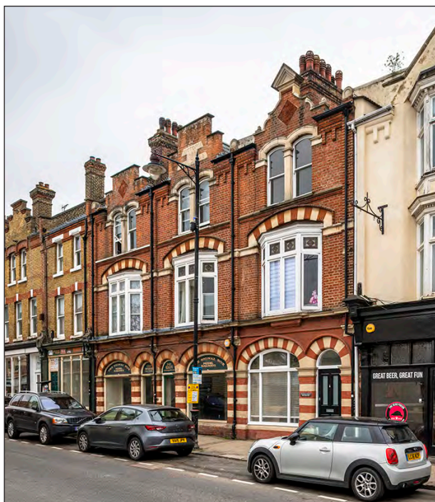
Fig. 32 Victoria Buildings, Nos 354-358 High Street Rochester [Chris Redgrave ©Historic England Archive, DP289270]
