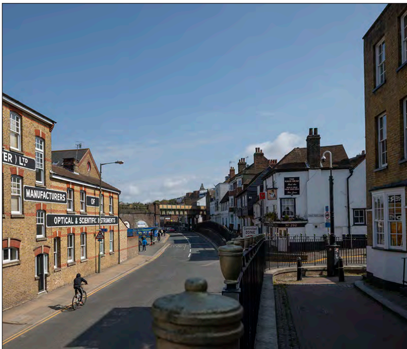
Fig. 82 The west end of Chatham Intra from the raised pavement of St Margaret's Banks in 2021 [Chris Redgrave ©Historic England Archive, DP289300]
