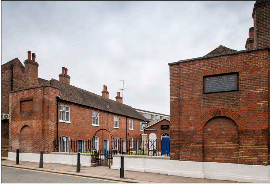
Fig. 45 The front elevation of the Sir John Hawkins' Hospital in 2021 [Chris Redgrave ©Historic England Archive, DP289356]
