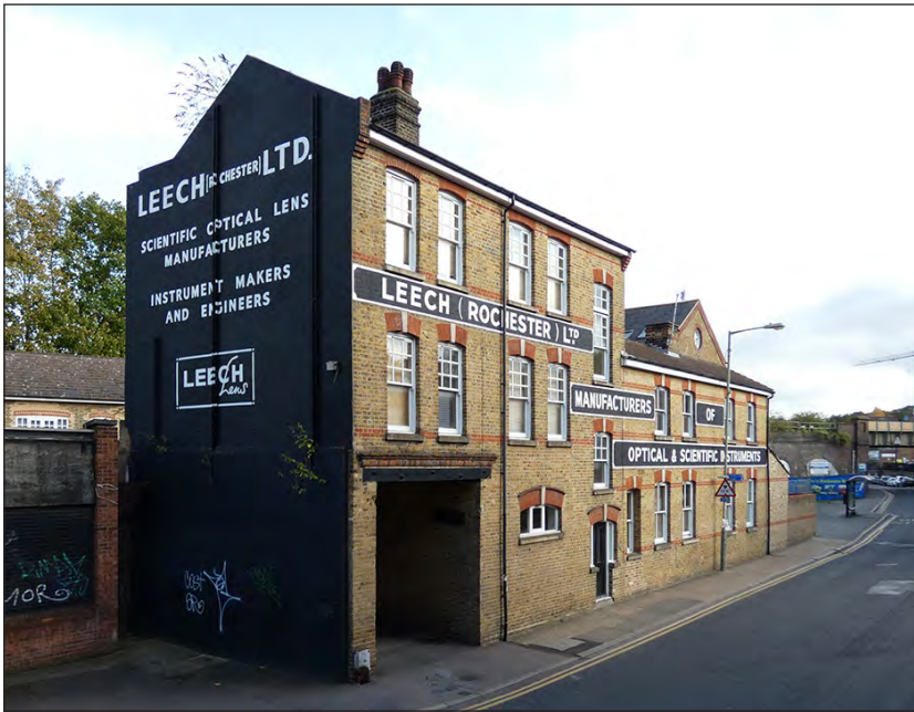
Fig. 92 Nos 273-5 Rochester High Street from the south west in 2021 [Joanna Smith ©Historic England, HSLSE09/P10]
