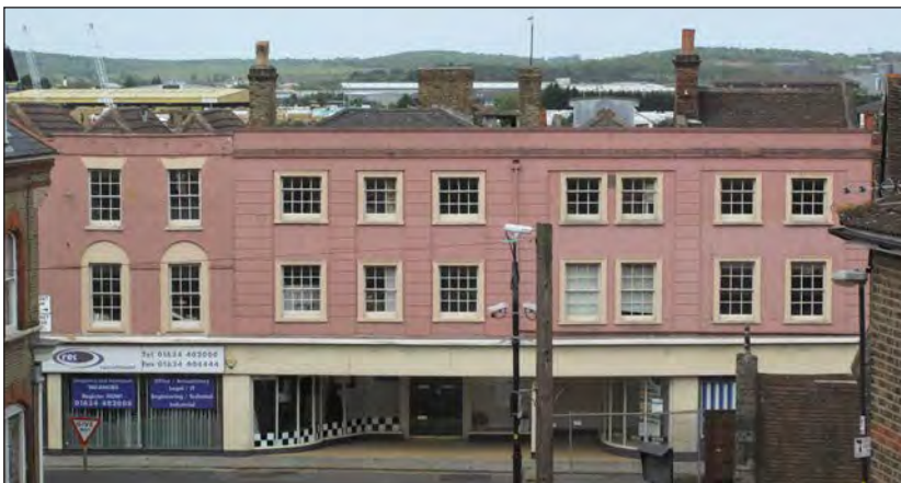
Fig 47 Nos 371-377 High Street Rochester viewed from Gundulph Road in 2004 [Jonathan Clarke ©Historic England HSLSE09/P3]
