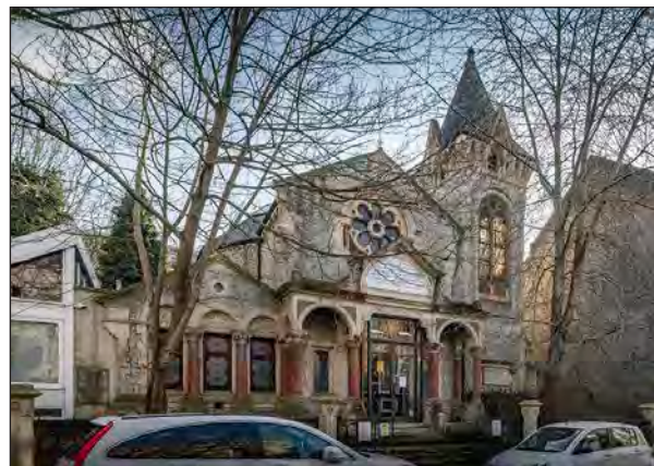
Fig. 117 Front elevation of Chatham Memorial Synagogue in 2021 [Chris Redgrave ©Historic England Archive, DP289272]
