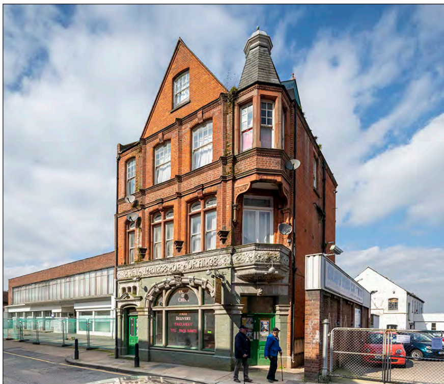
Fig. 107 The Prince of Orange public house, No. 21 Chatham High Street in 2021 [Chris Redgrave ©Historic England Archive, DP289359]
