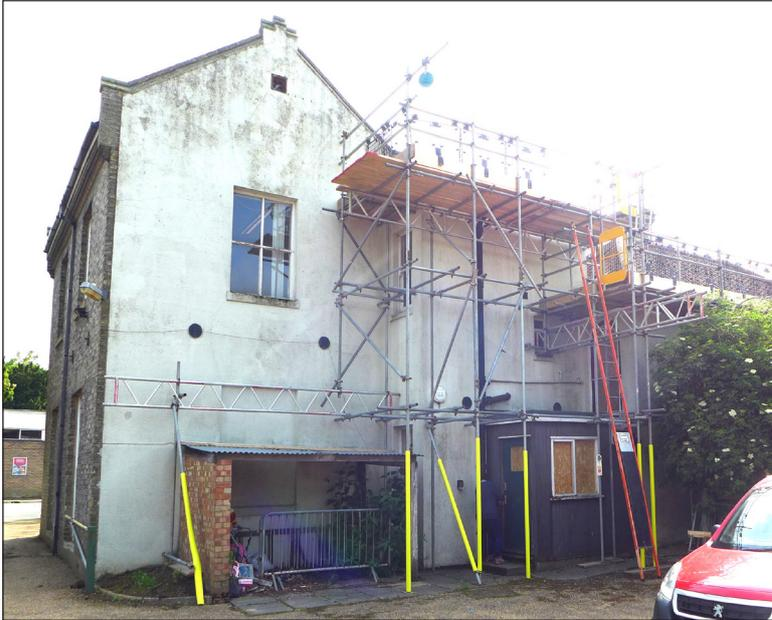
Fig. 44: Photograph of 2021 showing the rendered north elevation of the Victorian east extension. Modern alterations include the blocking of the ground-floor window and addition of a single-storey porch (right; since demolished). [James Shemmonds © Historic England]
