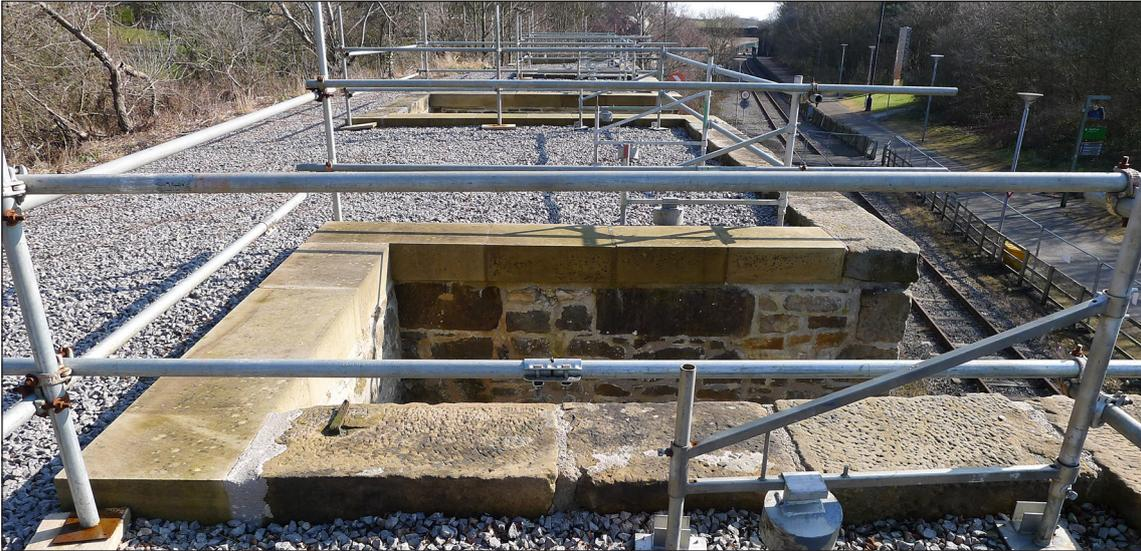
*Figure 13. Coping stone (with part of an iron strap) wrongly re-sited to the north-west corner of bay II. Note the large padstones surviving in the top of the far wall. [Marcus Jecock 6 March 2020 © Historic England].*
