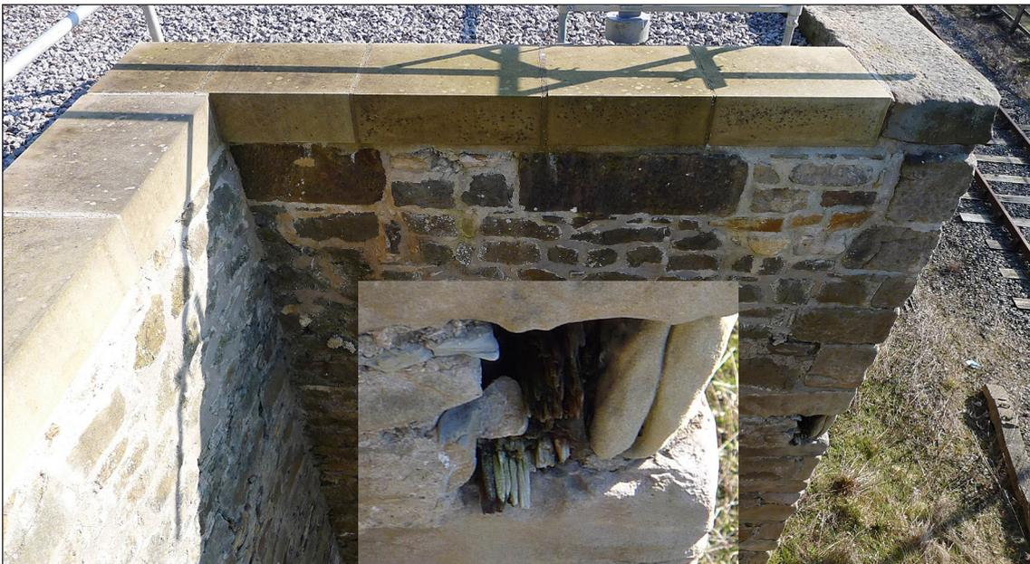
Figure 16. Socket in the east wall of bay II for tying the hopper support-framework to the bay wall. Inset: detail of surviving *in-situ* timber. [Marcus Jecock 6 March 2020 © Historic England].
