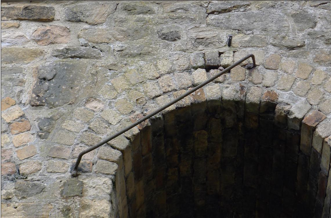
*Figure 21. Detail of metal hand rail attached to the arch rings in recess 45. [Marcus Jecock 6 March 2020 © Historic England].*
