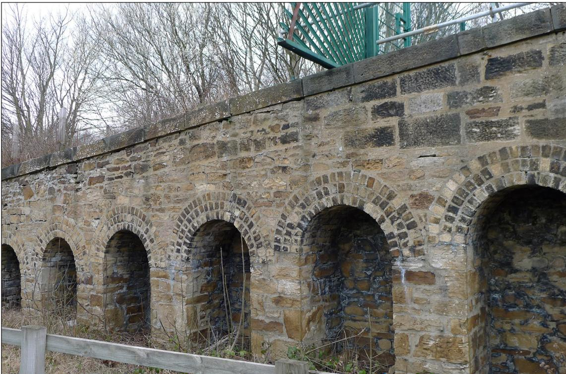
*Figure 9. The vertical raise in height to the Drops, destroyed by later rebuilding (the larger blocks at right of frame) east of the start of recess 10. [Marcus Jecock 6 March 2020 © Historic England].*
