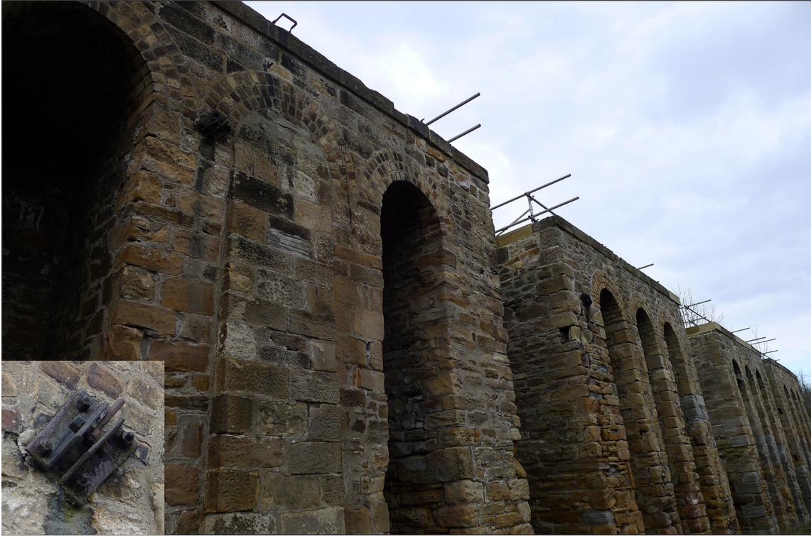
*Figure 23. Iron brackets either side of bay II, probably anchor points for cable-stays bracing an overhead power gantry. Inset: detail of western bracket showing end of in-situ cable. [Marcus Jecock 6 March 2020 © Historic England].*
