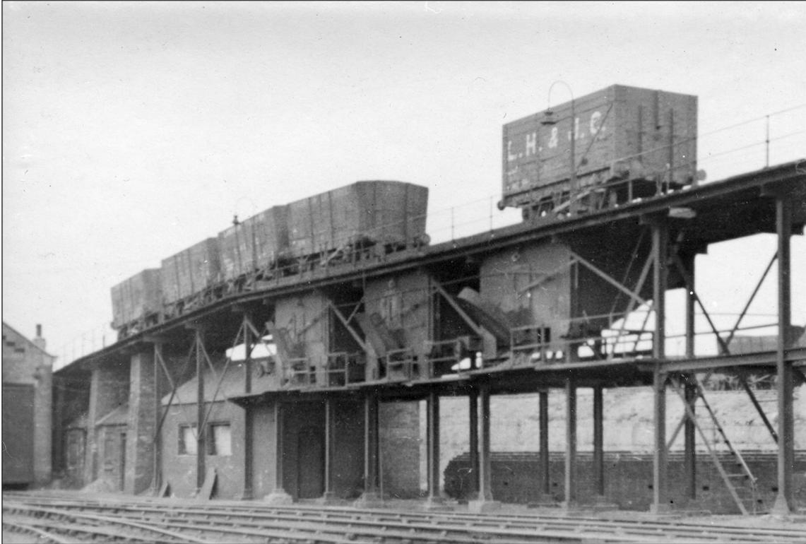
*Figure 27. The Lambton Railway's Philadelphia coaler as photographed on 2 July 1938. Note the stone piers to the ramped section and the metal bunkers with chutes that hinged up out of the way when not in use. [Unknown photographer; © Ken Hoole Collection/Head of Steam – Darlington Railway Museum].*
