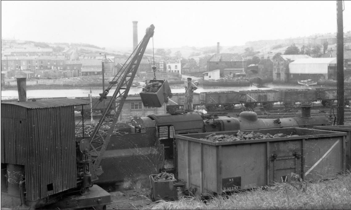
*Figure 31. Steam crane coaling a locomotive tender at Whitby shed, in August 1957. [NERA Collection, reproduced with permission].*
