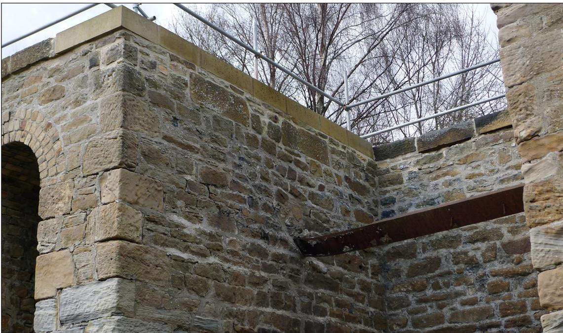
*Figure 14. Padstones in the west wall of bay III. The narrow stone fillet and the coping stones above the two large in-situ padstones represent modern 'over-restoration'. [Marcus Jecock 6 March 2020 © Historic England].*
