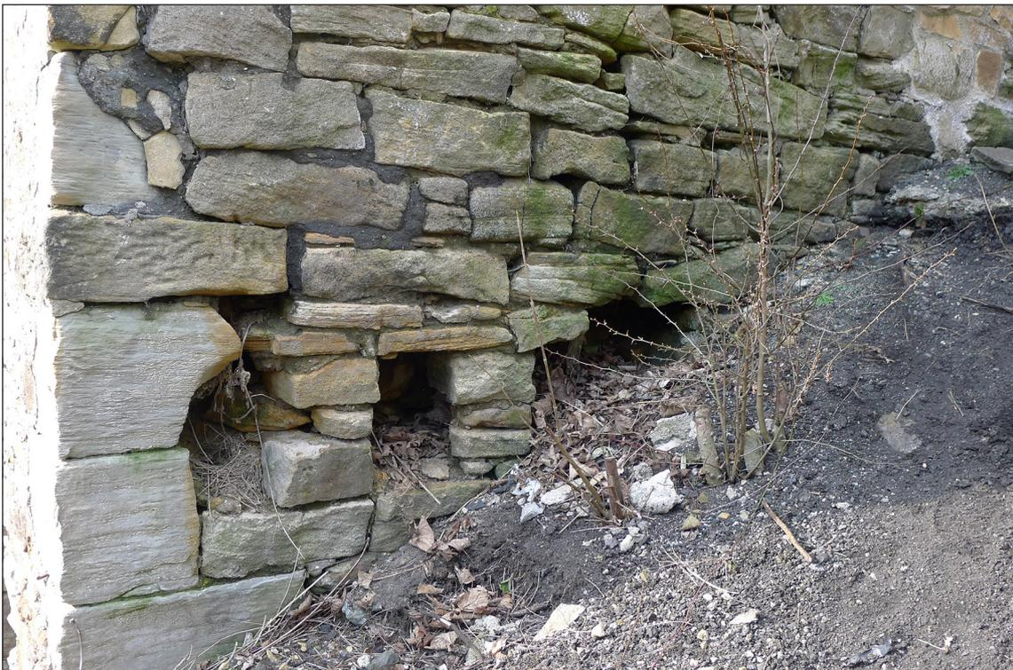
Figure 20. Joist sockets in the west wall of the demolished bay V. [Marcus Jecock 6 March 2020 © Historic England].
