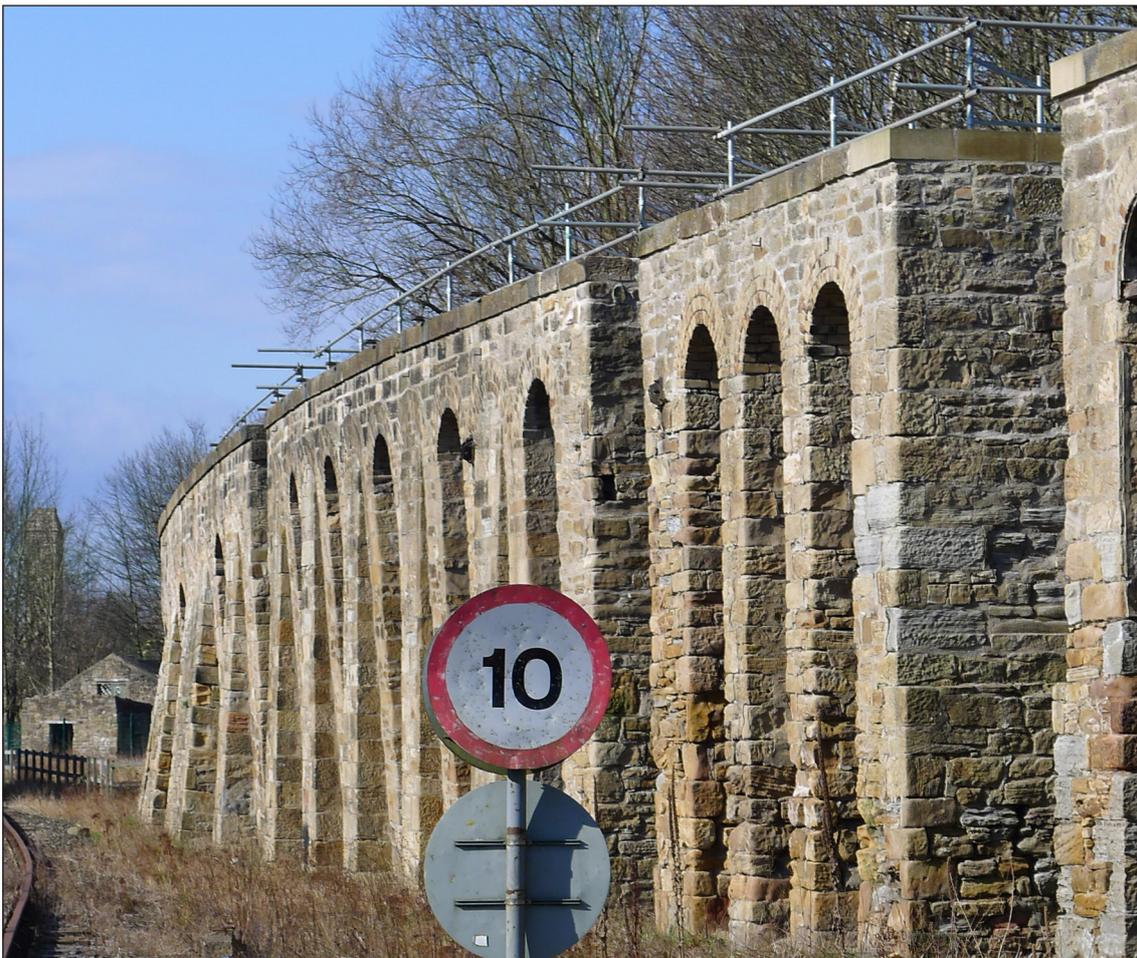
*Figure 10. The Drops looking west from bay IV, showing the lean out of the curved ramp section and the buttressing added to remediate the lean. [Marcus Jecock 6 March 2020 © Historic England].*
